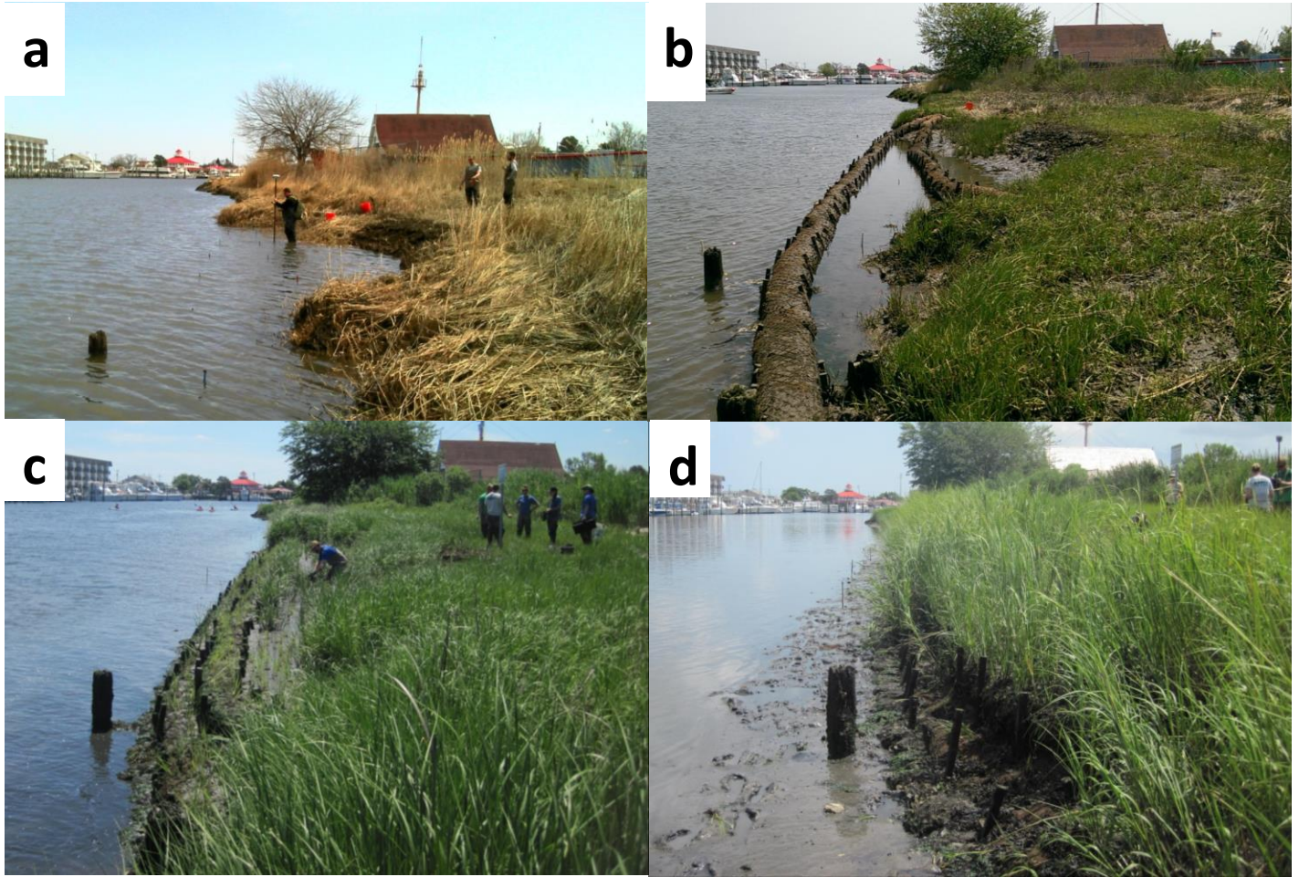
Figure D1. Time series for Lewes Marsh site living shoreline looking southeast: a) pre-installation, April 2014; b) post-installation June 2014; c) June, 2015; d) August, 2016.
