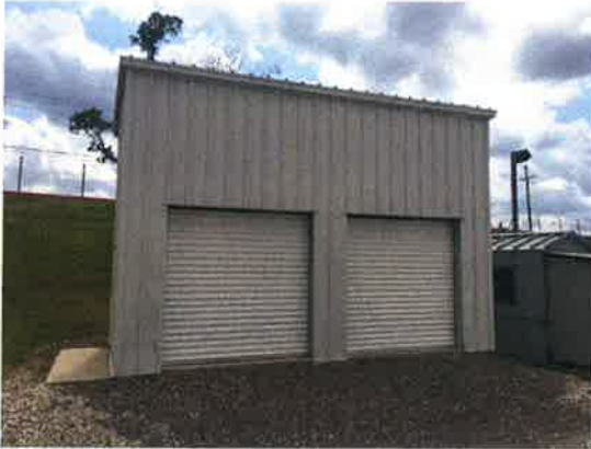
Similar metal building – NJ facility
