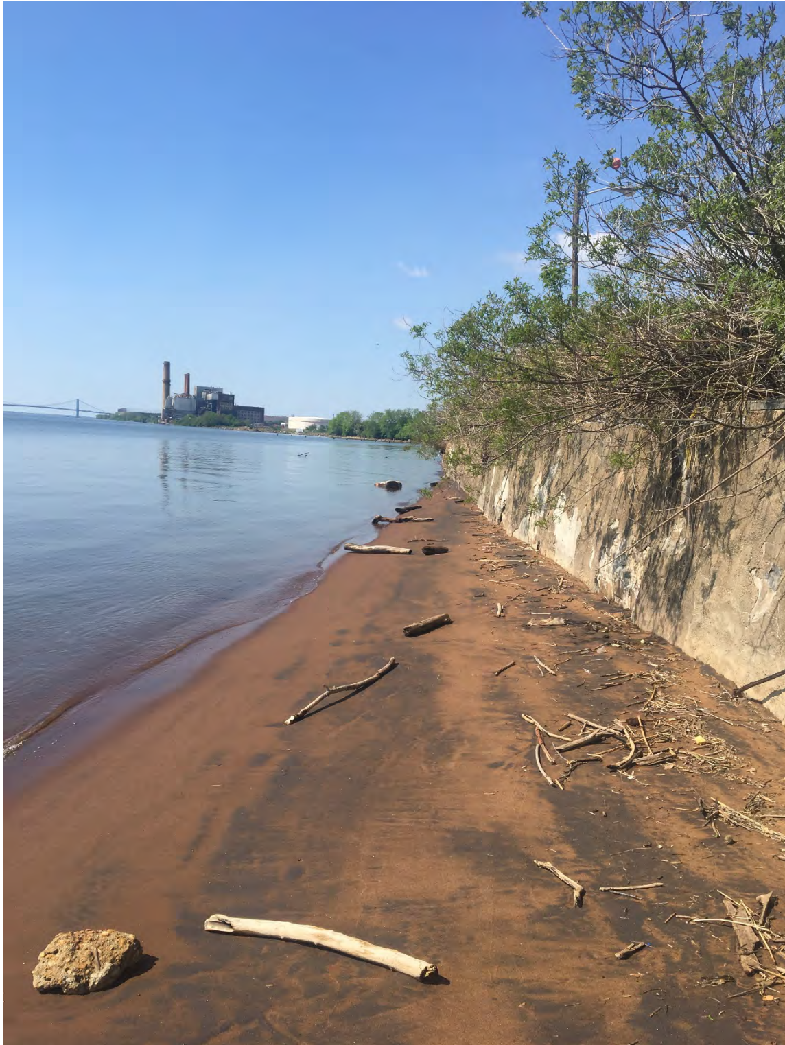
Photograph 3 – View of seawall along the Delaware River, looking south. Drift deposits along the seawall depict the approximate location of the Mean High Waterline.
