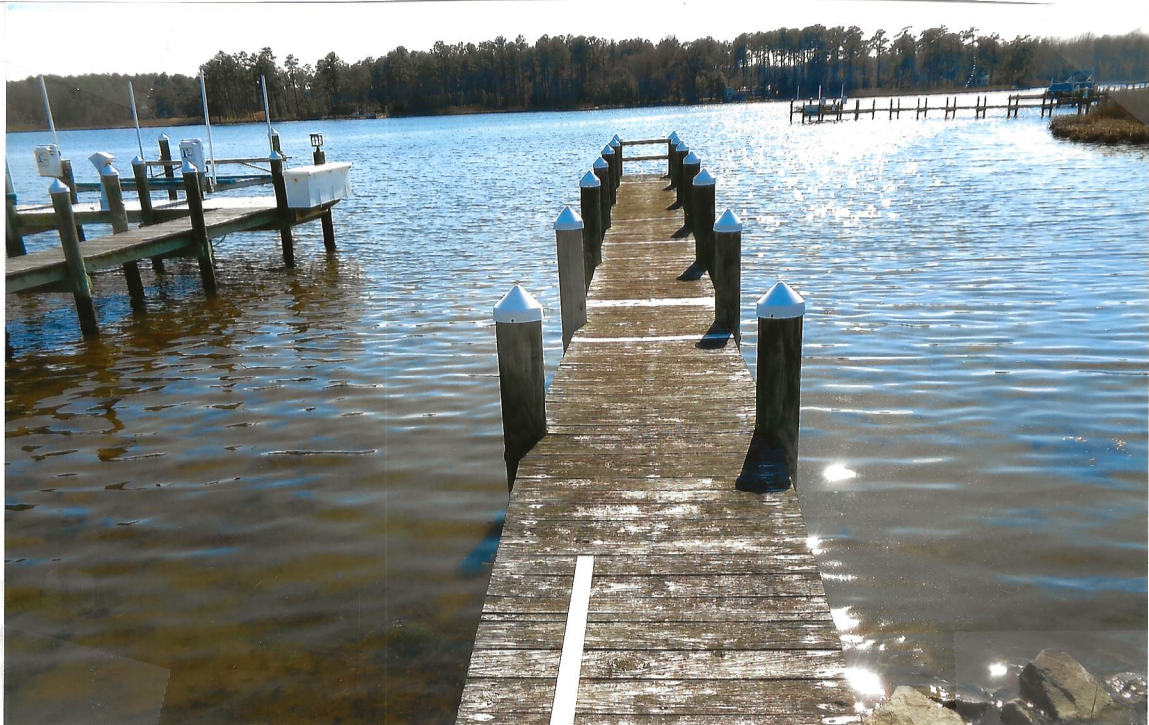
Figure 6. Aerial (top) and ground-level (bottom) photographs of site, 34477 Skyler Drive, Lot 48, The Villages at Herring Creek, Lewes, Sussex County, Delaware. Existing 80' x 3' wetland walkway (over Federal wetlands) and 70' x 4' pier present (authorized by SL-144/07, Harold Dukes, Jr., lessee). SU-223-10 authorizes owners of Lots 49 and 50 to use the structure. Applicant proposes to extend pier by adding a 10' x 4' fixed pier, a 10' x 3' gangway, and a 25' x 6' floating pier. See Figures 7 and 8 for plan view and cross-section (prepared by applicant).
