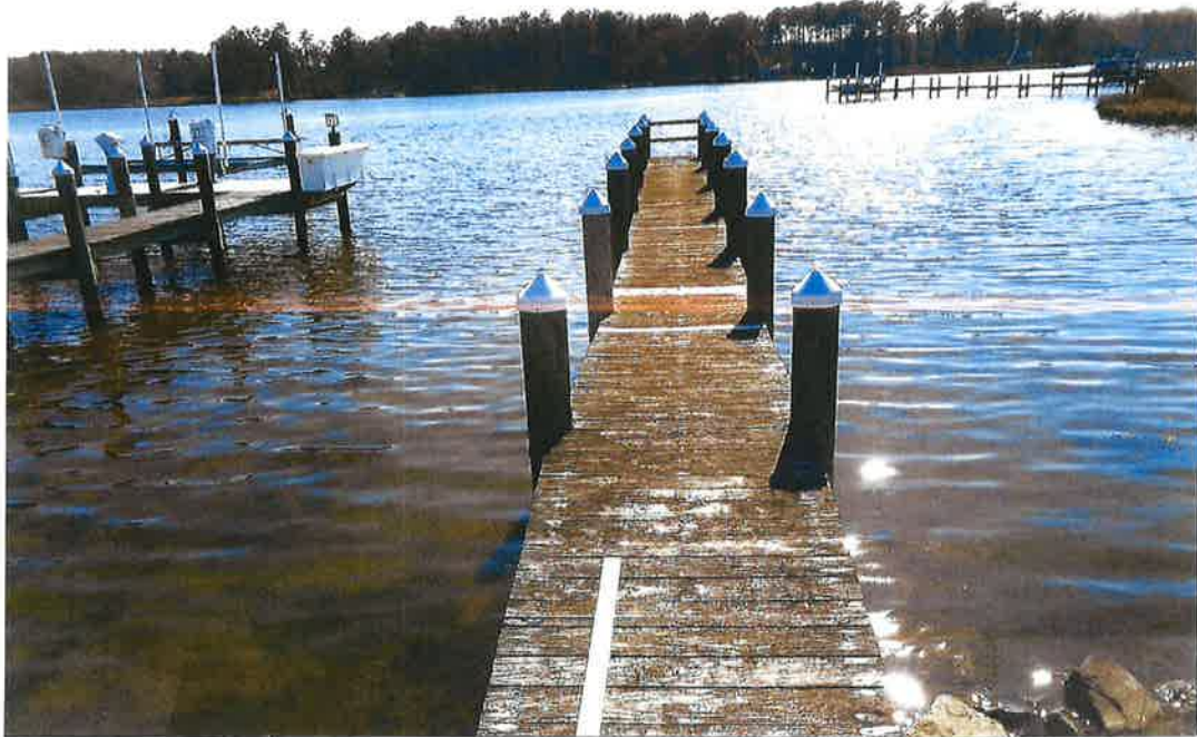
Figure 6. Aerial (top) and ground-level (bottom) photographs of site, 34477 Skyler Drive, Lot 48, The Villages at Herring Creek, Lewes, Sussex County, Delaware. Existing 80' x 3' wetland walkway (over Federal wetlands) and 70' x 4' pier present (authorized by SL-144/07, Harold Dukes, Jr., lessee). SU-223-10 authorizes owners of Lots 49 and 50 to use the structure. Applicant proposes to extend pier by adding a 10' x 4' 45'x4' fixed pier and a 10' x 3' gangway, and a 25' x 6' a 12'x6' floating pier. See Figures 7 and 8 for plan view and cross-section (prepared by applicant).
