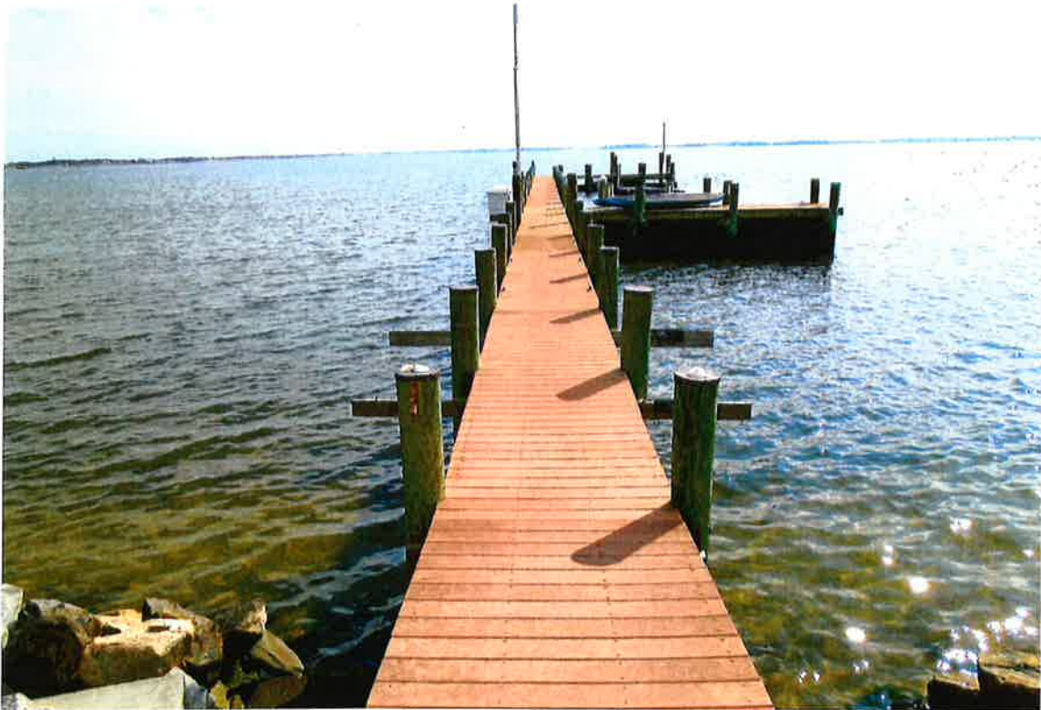
Figure 7. Photograph of site, 318 Salisbury Street, Seabreeze, Dewey Beach, Sussex County, Delaware (Tax Map Parcel #3-34-20.17-14.00), adjacent to Rehoboth Bay. Existing structures, 110' bulkhead; 110' stone rip-rap; 170' x 4' pier; two 6' x 30' docks; 4-piling boat lift; and floating PWC dock authorized by SL-065/05; SU-376/06; and SU-022/13. Applicant proposes to install a 12' x 4' gangway and a 6' x 25' floating dock. See Figure 8 for plan view and cross-section sketches.
