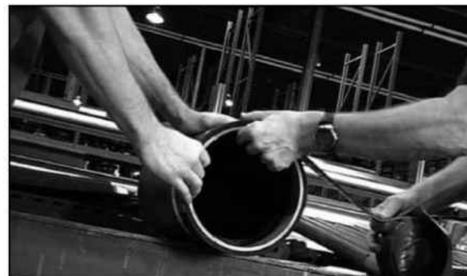
STEP C: Repeat steps A and B on the opposite side of the valve to ensure uniformity of the CheckMate's® O.D. is consistent and matches the pipe I.D.
