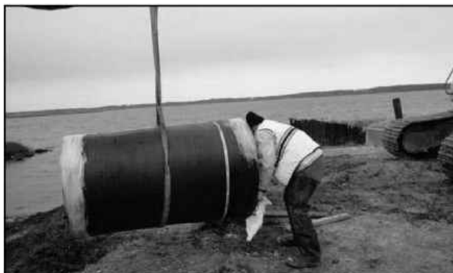
STEP D: Lubricate the valve and rubber adhesive strip surface. Slide valve into pipe. Ensure the area marked TOP is in the 12:00 position.
