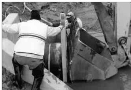
Pallet Push method for installing CheckMate® Valve
