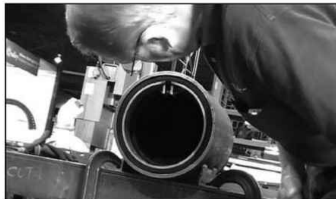
STEP E: Check O.D. of the valve to ensure it fits snugly into the I.D. of pipe. If loose, add another layer(s) of the rubber adhesive strip.
