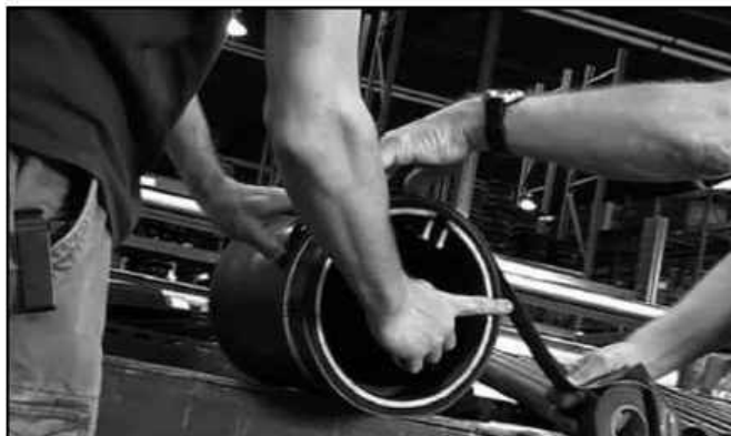
STEP B: Slowly rotate the valve while firmly pressing the rubber adhesive strip onto itself in concentric layers until valve O.D. is equal to or a fraction smaller than pipe I.D.
