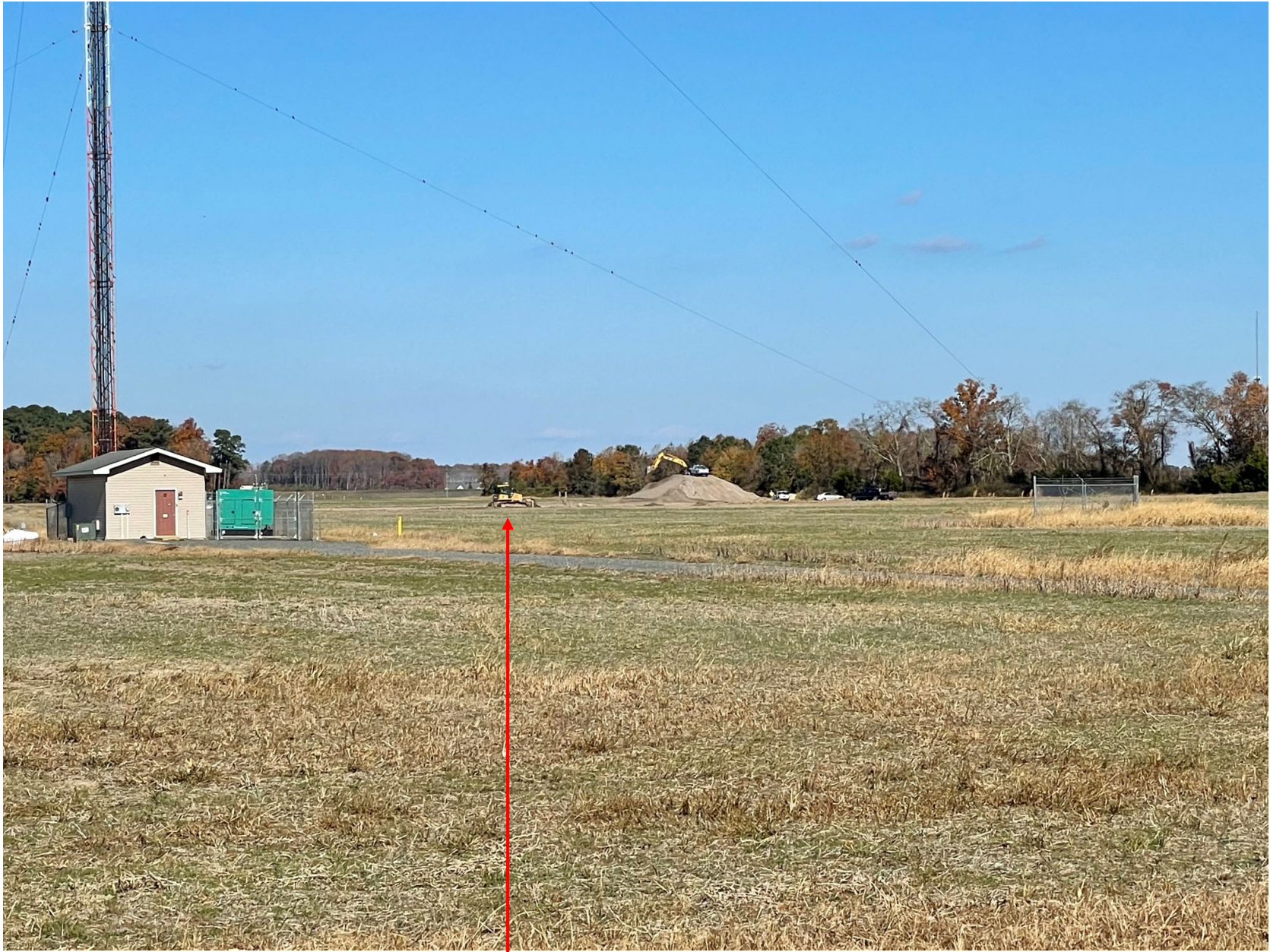
Dirt being excavated
