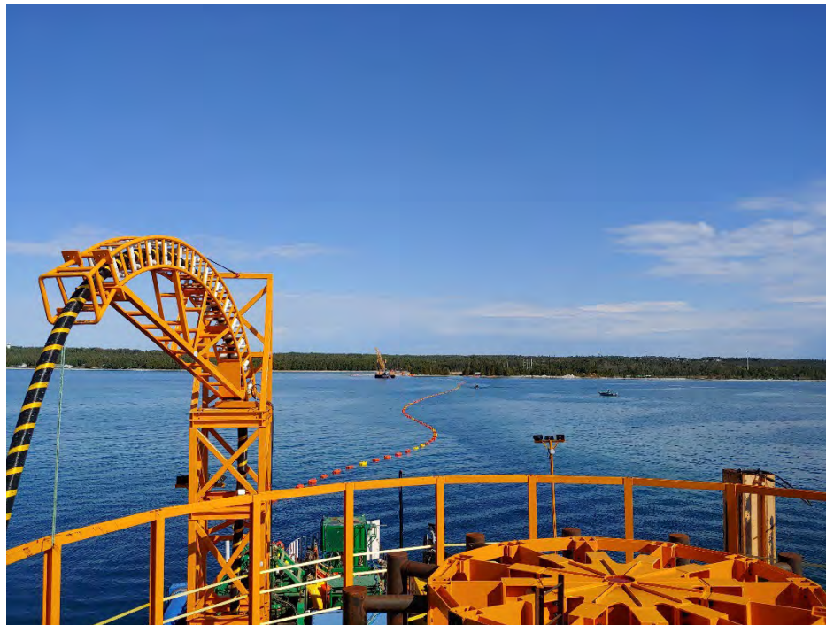
Figure 2-6. Example of Shallow Water Cable Installation
