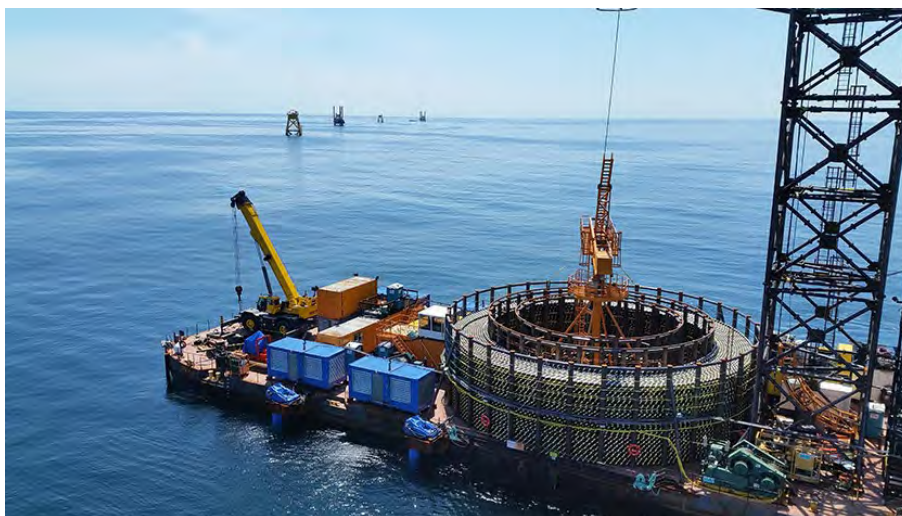
Figure 2-5. Block Island Cable Installation Source: www.oceannews.com
