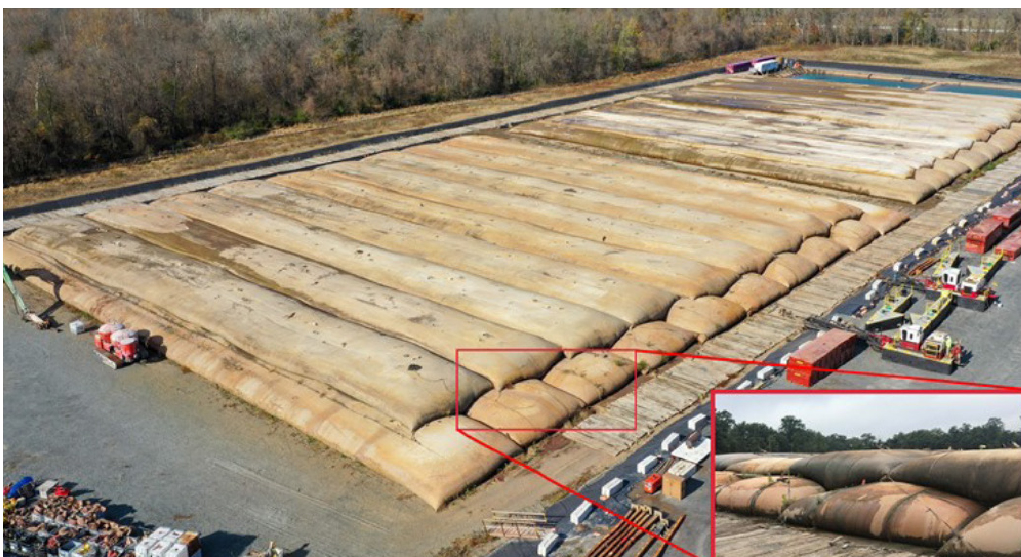
This image shows an example of a Passive Dewater Operation using Geobags.
