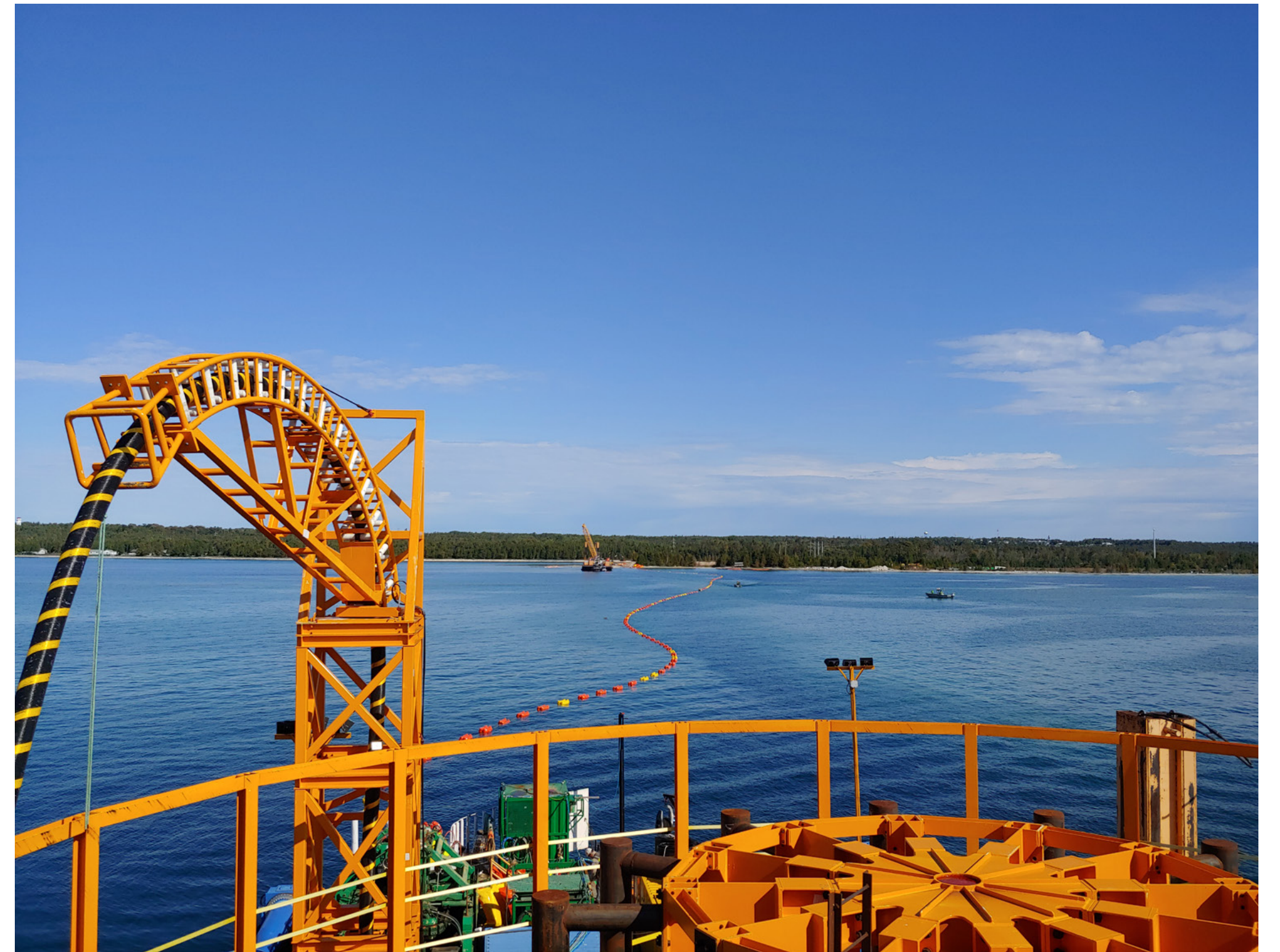
This image shows an example of Shallow Water Cable Installation.
