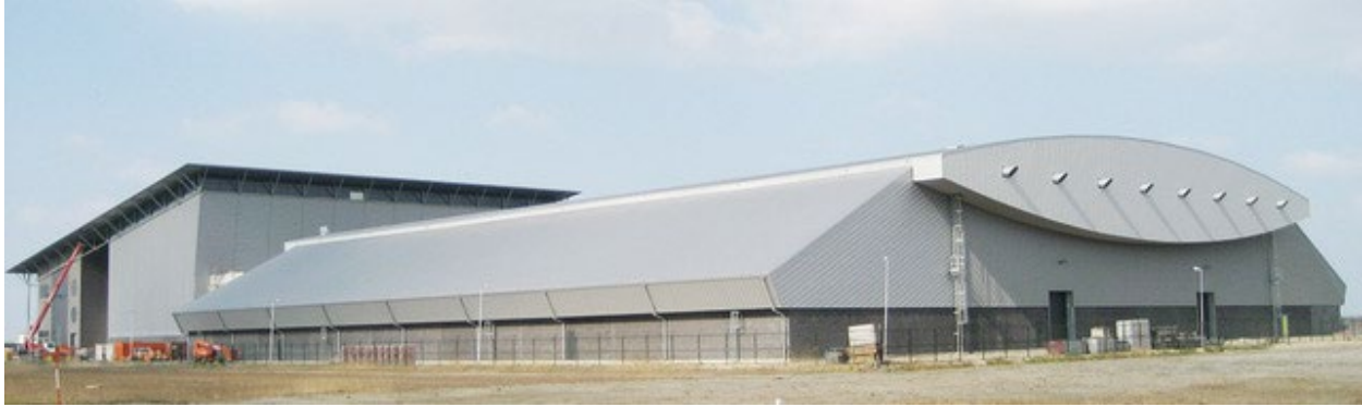
Figure 3.3-1. DC to AC power conversion building for 700 MW HVDC Norend cable between Norway and the Netherlands
