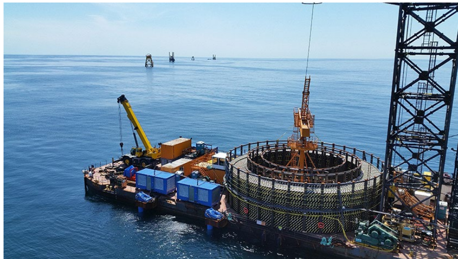
Figure 2.1-13. Block Island Cable Installation Source: www.oceannews.com
