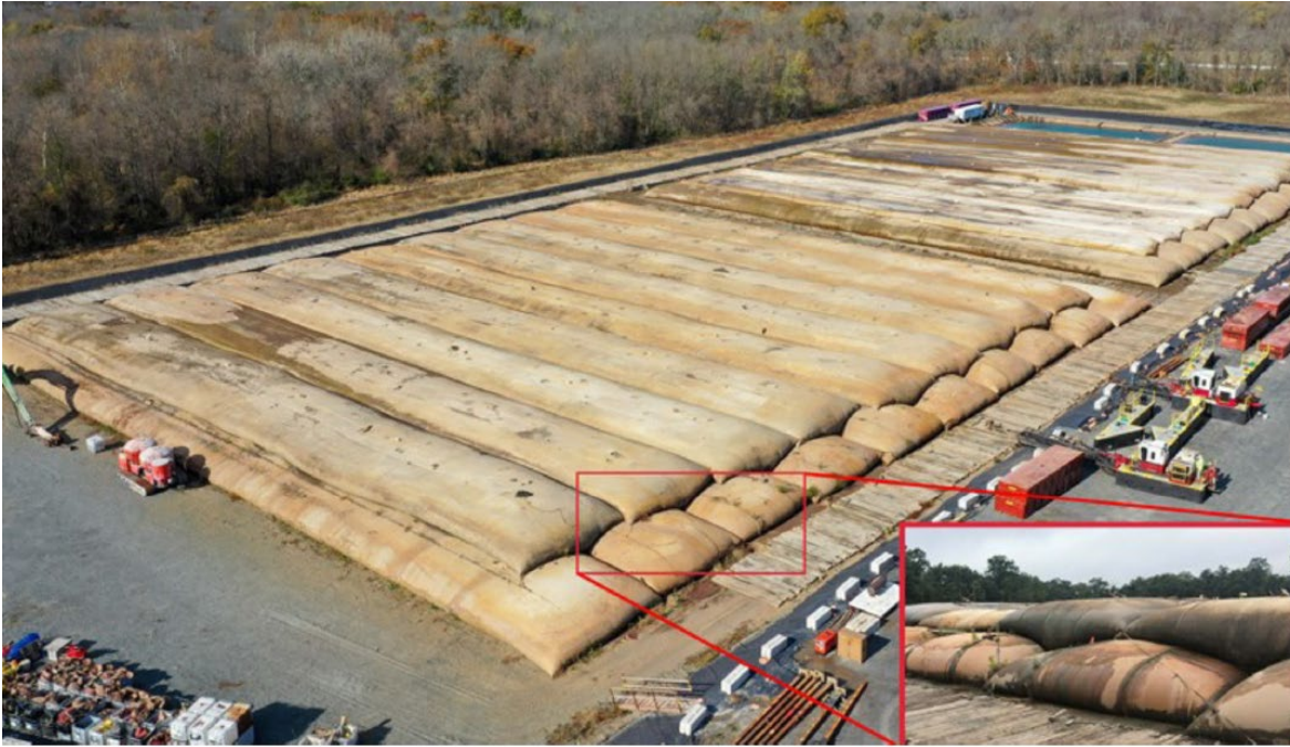
Figure 2.1-18. Example of a Passive Dewater Operation using Geobags
