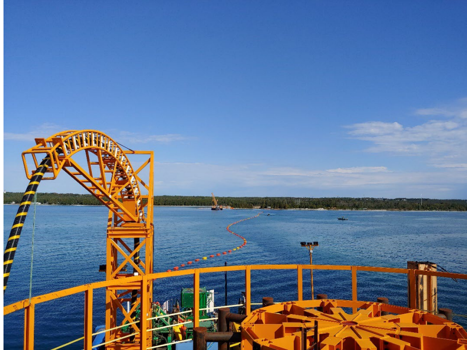
Figure 2.1-14. Example of Shallow Water Cable Installation
