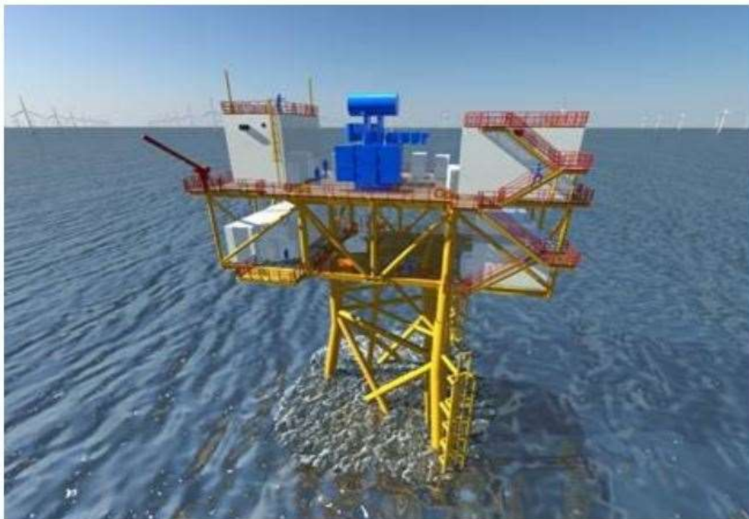
Figure 3.1-7. OSS on Jacket Foundation (Source: HSM Offshore)
