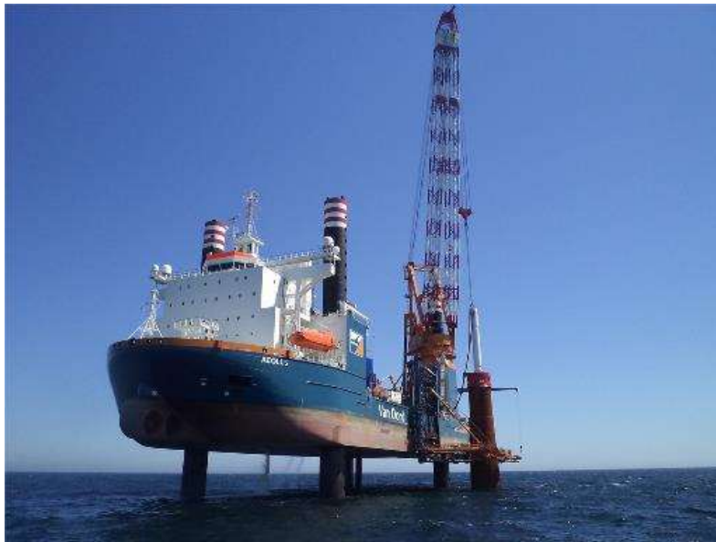
Figure 3.2-2. Monopile Installation (Source: Globalenergyworld.com)
