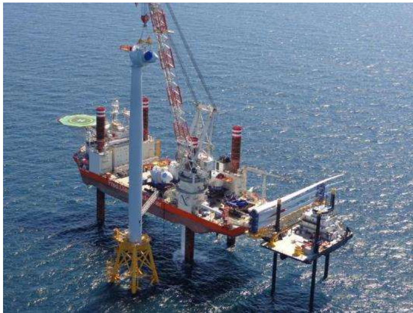
Figure 3.2-14. Offshore WTG Installation Vessel (Source: blockisland.com)
