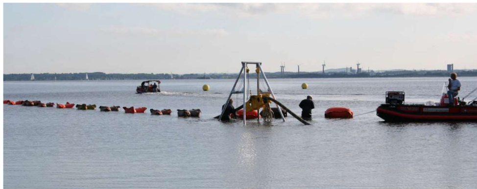
Figure 3.2-8 Example of Shallow Water Cable Installation
