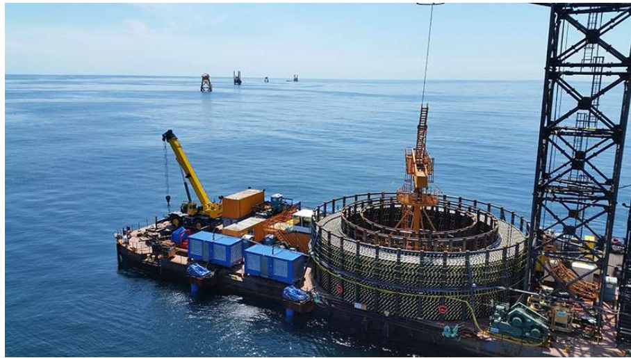
Figure 3.2-7. Block Island Cable Installation Source: www.oceannews.com
