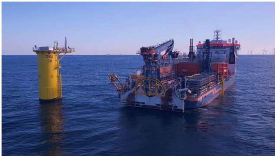
Figure 3.2-11. Dynamically Positioned Cable Installation Vessel (Source: Deutsche Bucht and Van Oord)
