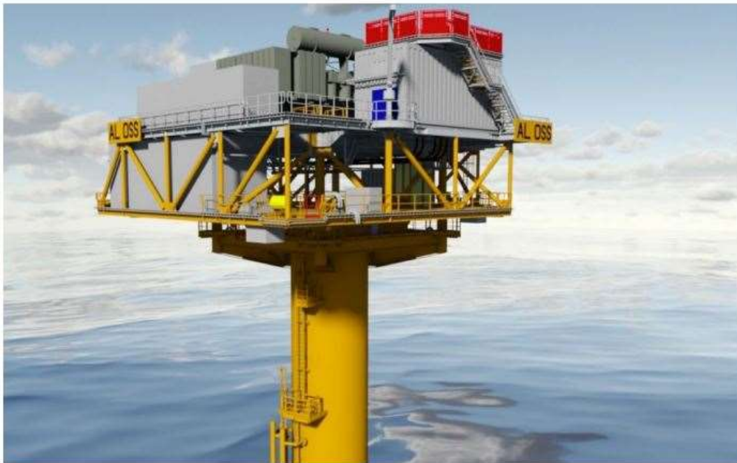
Figure 3.1-6. Design of Conceptual OSS atop a Monopile Foundation
