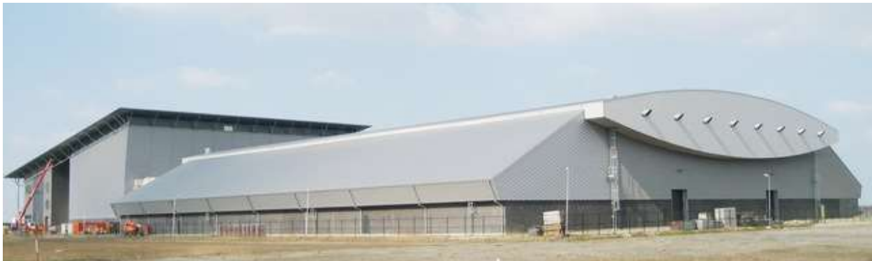
Figure 4.6-1. DC to AC power conversion building for 700 MW HVDC Norend cable between Norway and the Netherlands
