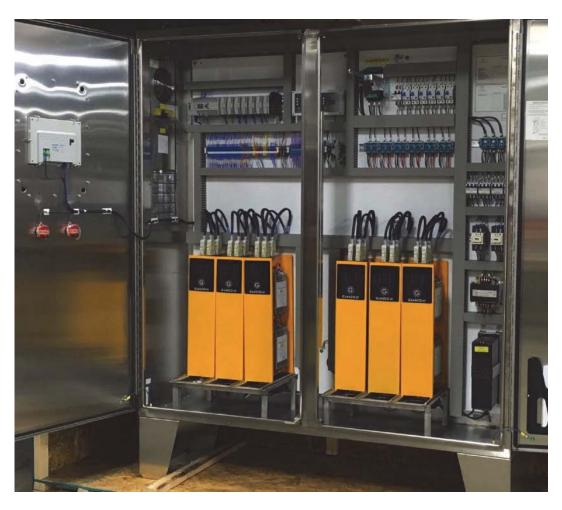
EXAMPLE OF THE INSIDE OF A BCC houses ballasts, UV meters, Disconnect Switches, Breakers, PLC, Lighting Contactors and other controls.
