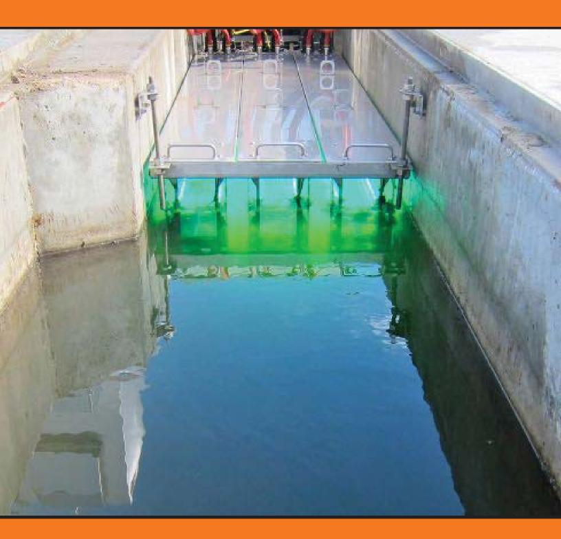
Horizontal Open Channel Ultraviolet Disinfection
