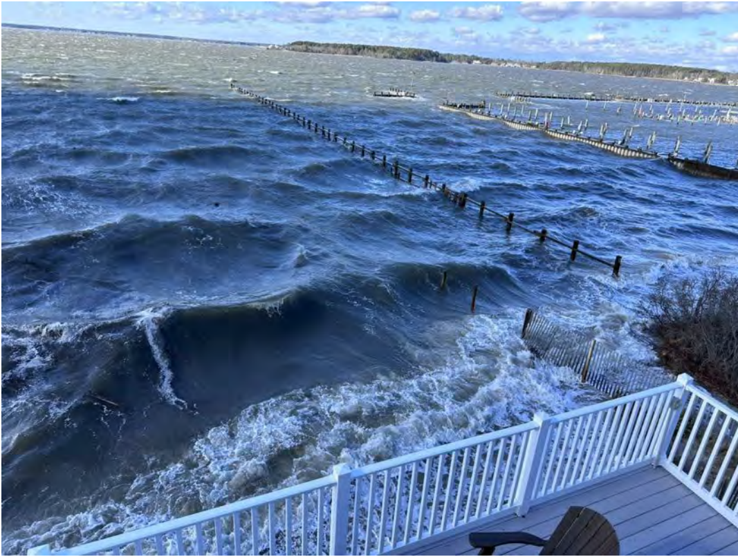
Looking down from the elevated deck during a recent storm event
