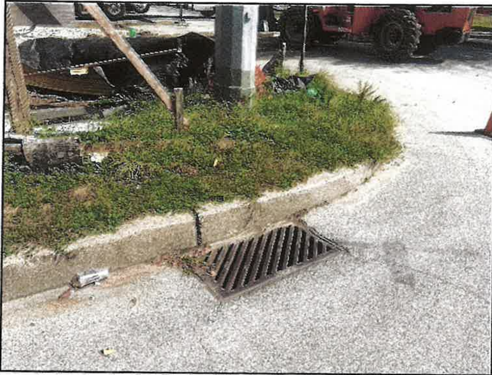
Photograph No. 3 Revised stormwater collection and concrete curb construction (439 Bradford Street)
