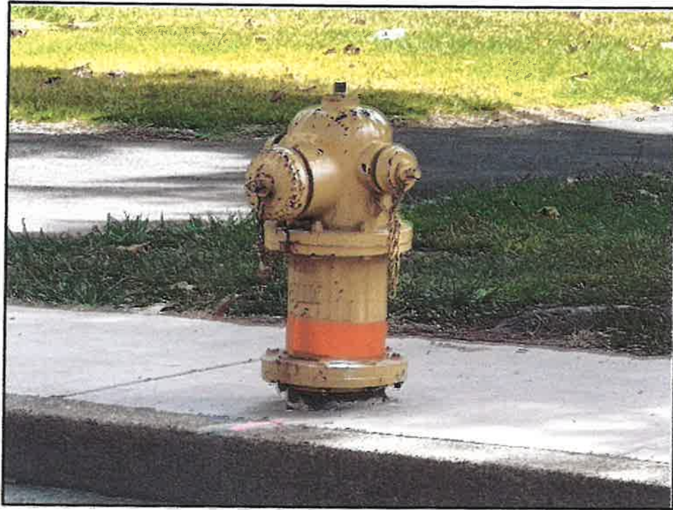
Photograph No. 5 Revised water service (439 Bradford Street)
