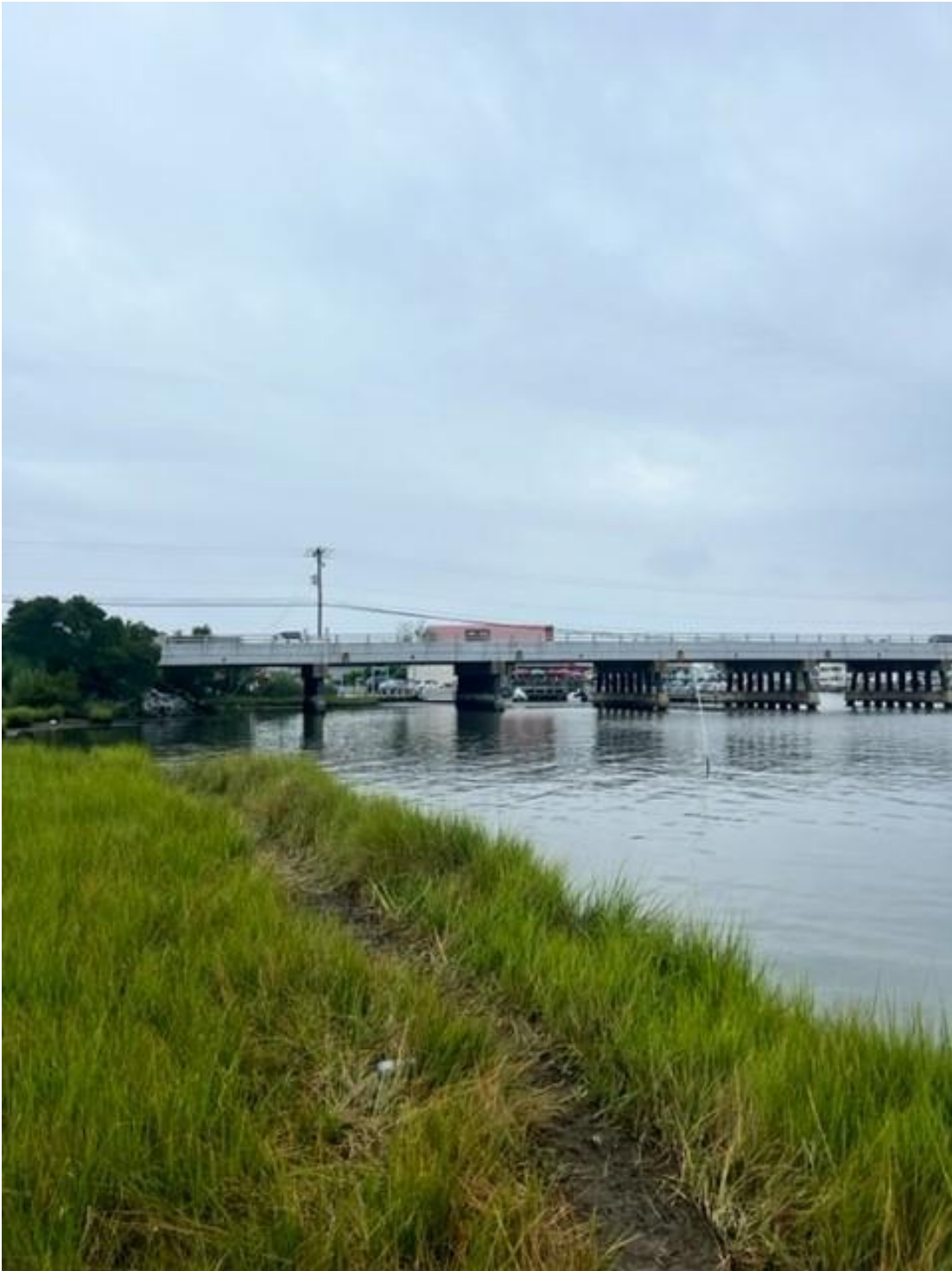
Photo 2: Looking south at BR 3-437 from northeast quadrant along The Ditch.
