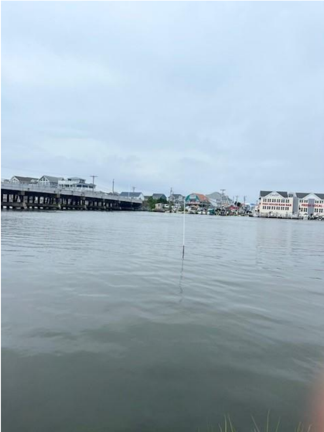
Photo 1: Looking west across The Ditch on the north side of BR 3-437.
