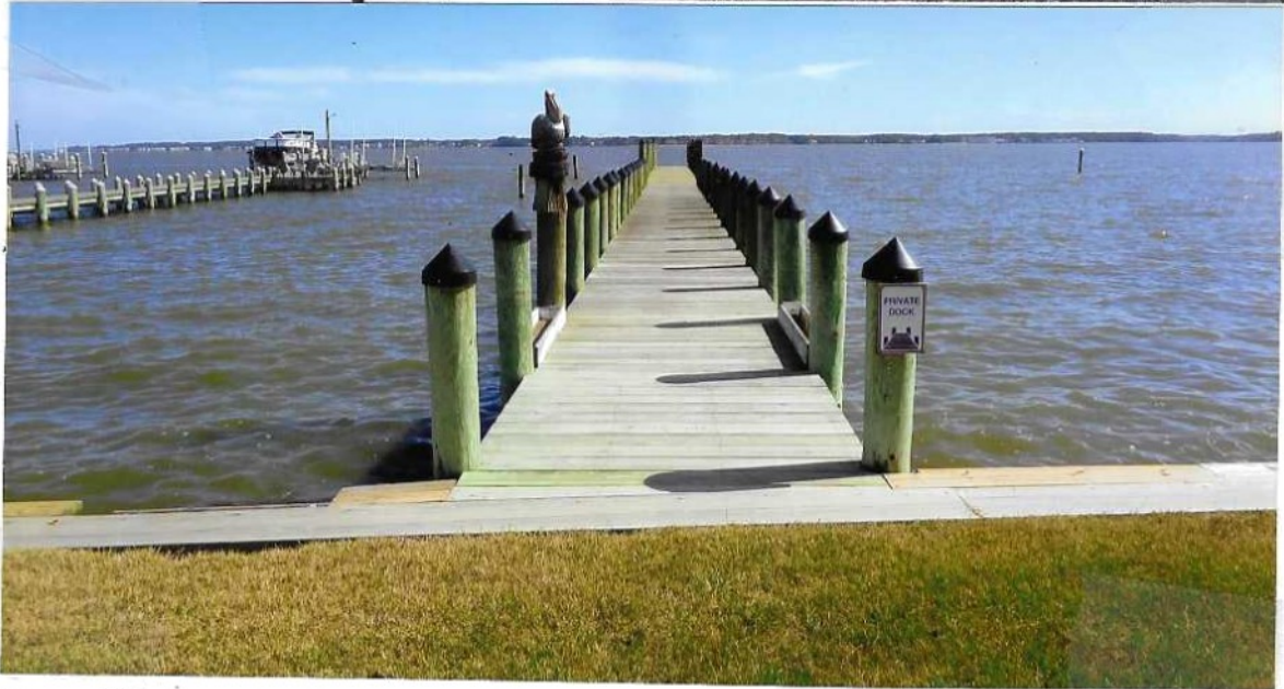
Figure 7. Photograph of project site, 33256 Mercer Avenue, Oak Orchard, Millsboro, Sussex County, Delaware (Tax Map Parcels #2-34-35.05-132.00 and 166.00), adjacent to Indian River showing existing pier (grandfathered), 104' long x 5.5' wide and 104' long x 6.5' wide (total length = 208'). Applicants propose to install a new 4-piling boat lift (12'6" C/C pilings) on the outer right side of the pier.
