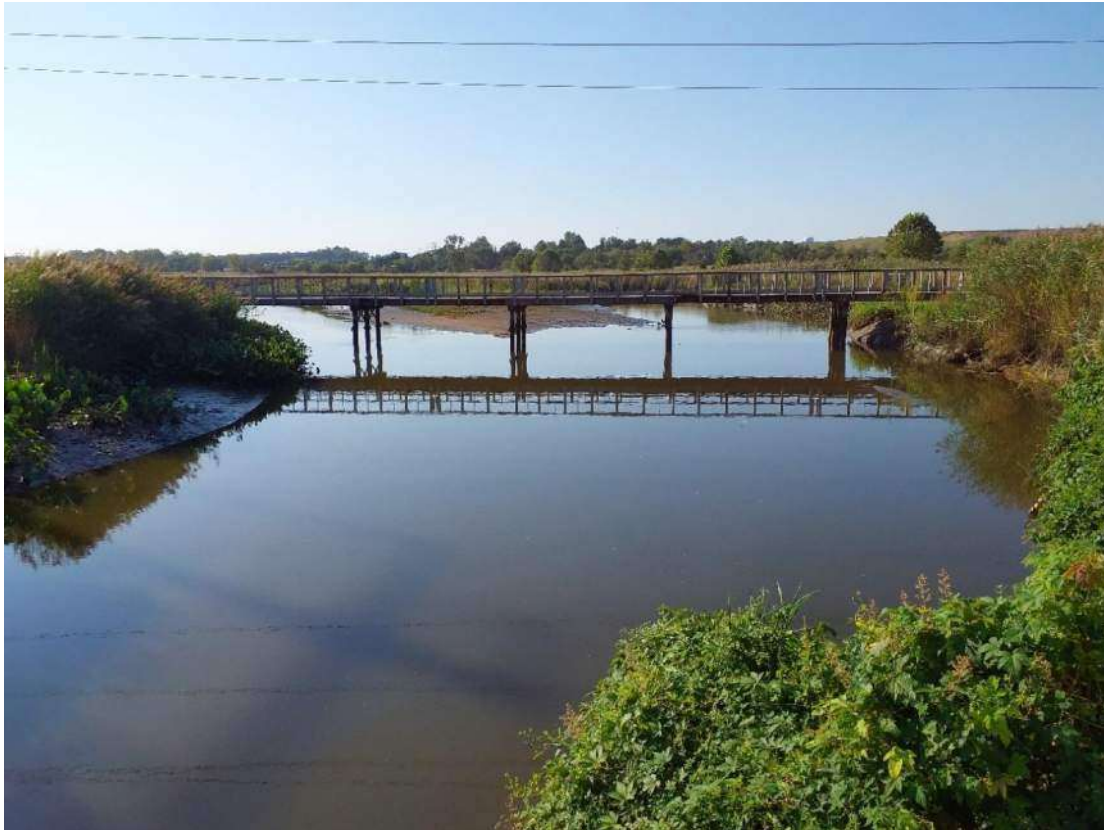
WC1: E1UBL3 watercourse (Little Mill Creek) facing downstream.
