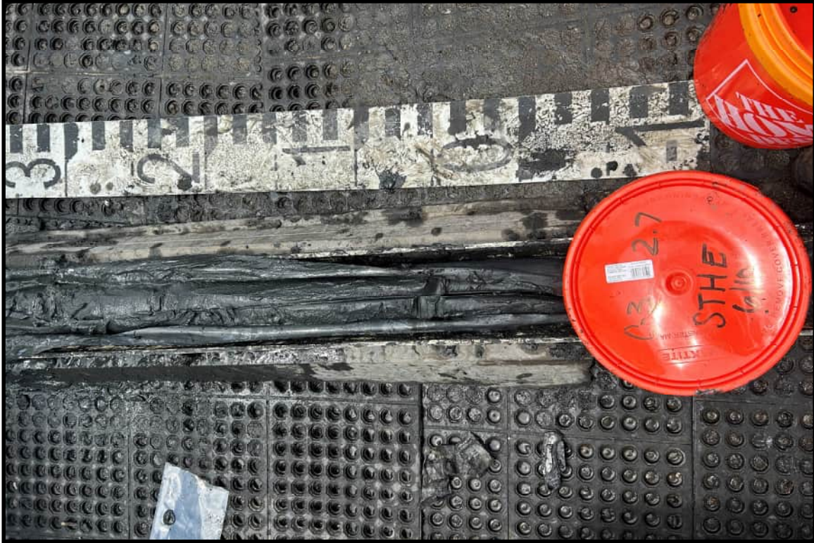
PHOTO No. 3: C-3 REQUIRED 2.7 FT.
