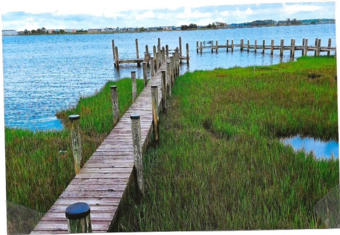
Figure 6. Ground level photograph of site, 806 S. Schulz Road, Fenwick Island, Sussex County, DE (Tax Map Parcel #134-23.16.-347.00), adjacent to Lighthouse Cove, Little Assawoman Bay, showing existing structure (left), an 80' long x 3' wide wetland walkway; 20' long x 3' wide pier; and 8' wide x 24' long dock. Applicants propose to remove existing 20' long x 3' wide pier and 8' wide x 24' long dock; and to construct a new 20' long x 4' wide pier; a 30' long x 4' wide pier extension; a 6' wide x 20' long dock; and a 4-piling 7-9K boat lift, and to obtain a new Subaqueous Lands Lease. New structure will not extend any farther channelward than neighbor's structure (right background). See Figure 7 for plan view and cross-section sketches.
