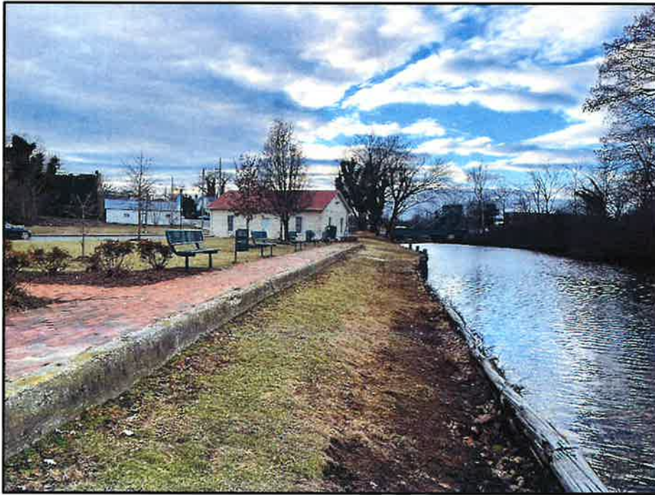
Photograph 3: View along the existing bulkhead looking west/downstream (January 2023).
