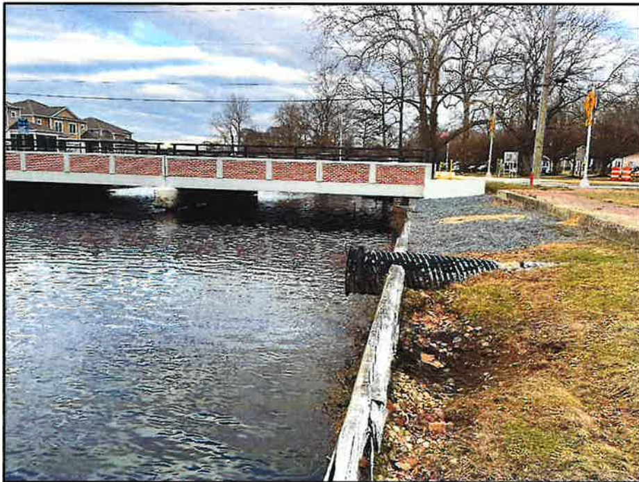
Photograph 1: View along the existing bulkhead looking east/upstream toward Delaware Ave (January 2023).
