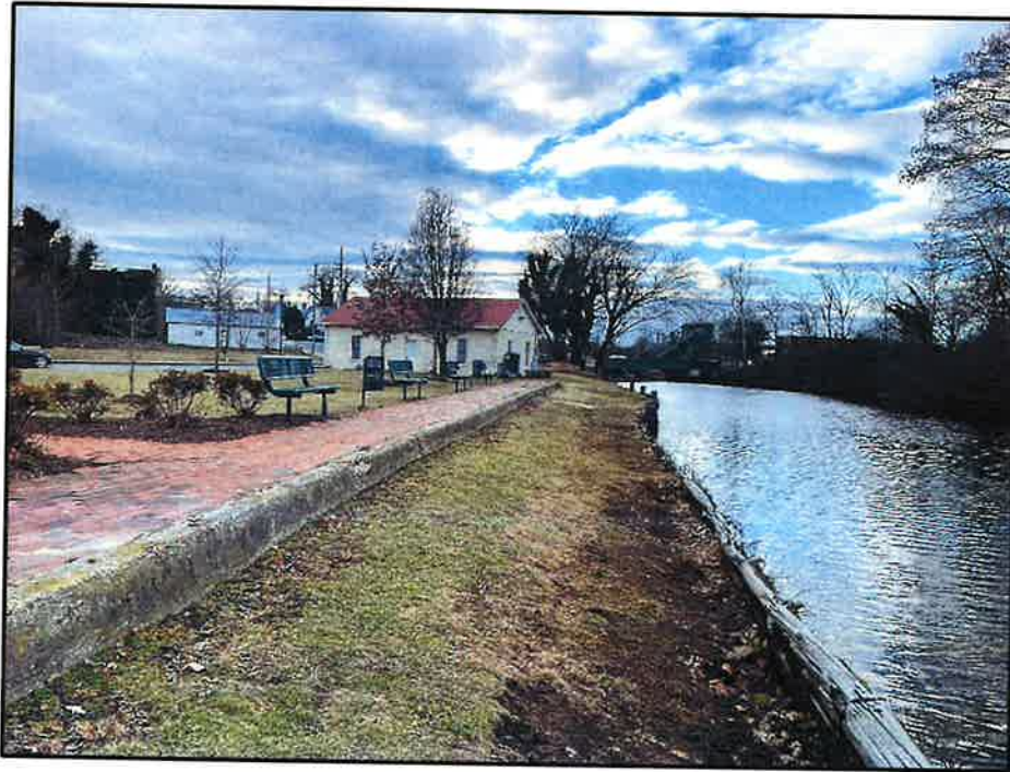
Photograph 3: View along the existing bulkhead looking west/downstream (January 2023).
