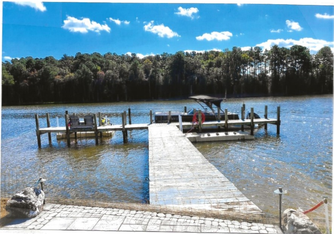
Figure 6. Photograph of project site, 39 Creek Drive, Winding Creek Village, Millsboro, Sussex County, Delaware, adjacent to Guinea Creek, showing existing structures (authorized by SL-374/20, copy included in application). Applicants propose to repair/replace existing 6' wide x 42' long pier and 6' wide x 54' long dock, and to install a new 4-piling boat lift. See Figure 7 for plan view and cross-section sketches.
