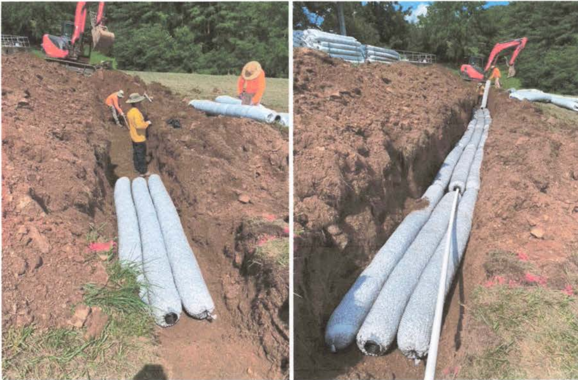
Trench installation showing EZ Flows being placed.
