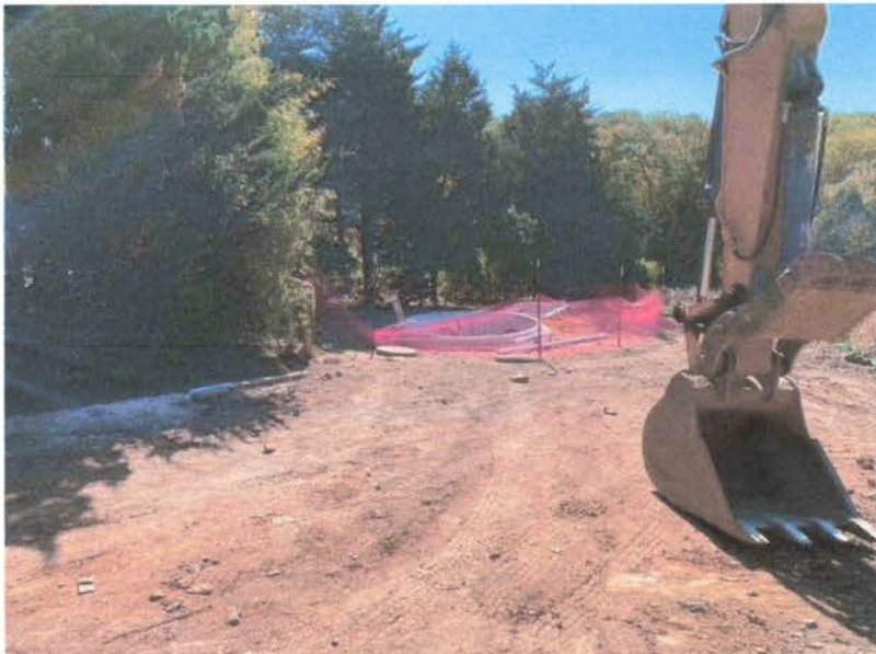
10/24/2023 Dosing Station under construction.
