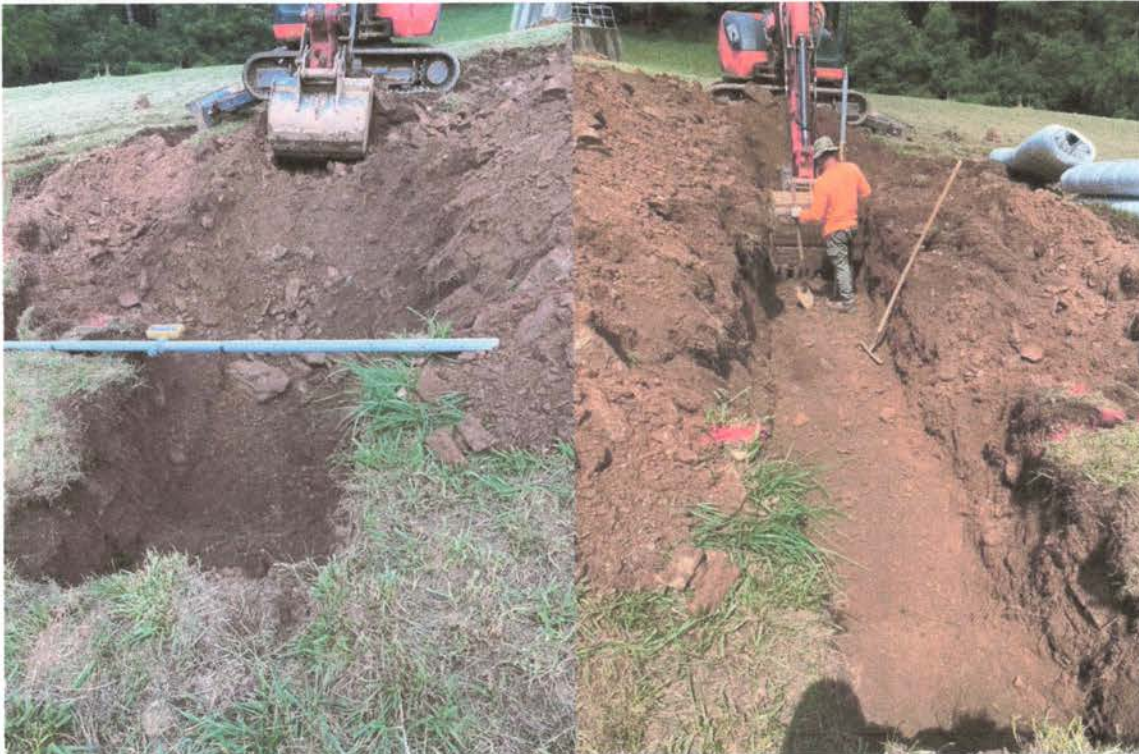
7/10/2023 Excavation of trench where trench #3 was planned.
