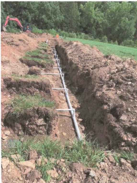
7/21/2023 Manifold installation (left). Trench #20 being installed (right).
