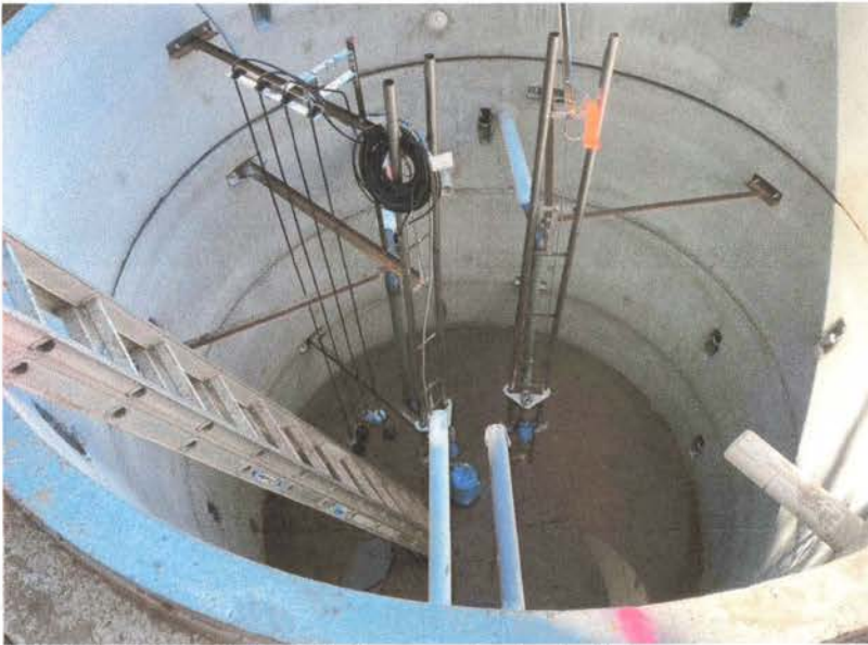
10/24/2023 Dosing Station under installation.
