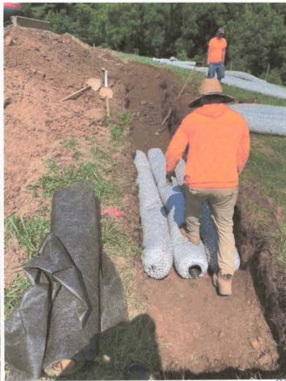
7/21/2023 Manifold installation (left). Trench #20 being installed (right).
