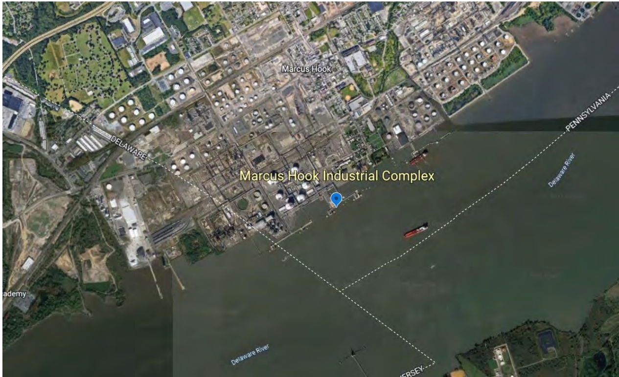
Figure 2: Aerial Photo of Marcus Hook Terminal (formerly Marcus Hook Industrial Complex) (Photo Courtesy Google Earth).
