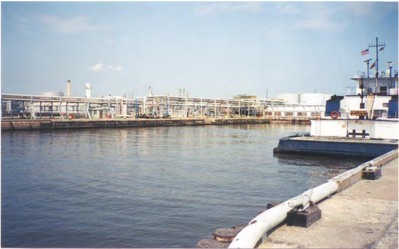
Figure 6: View of Marcus Hook Terminal Inner Barge Dock Berth 1B (looking west).
