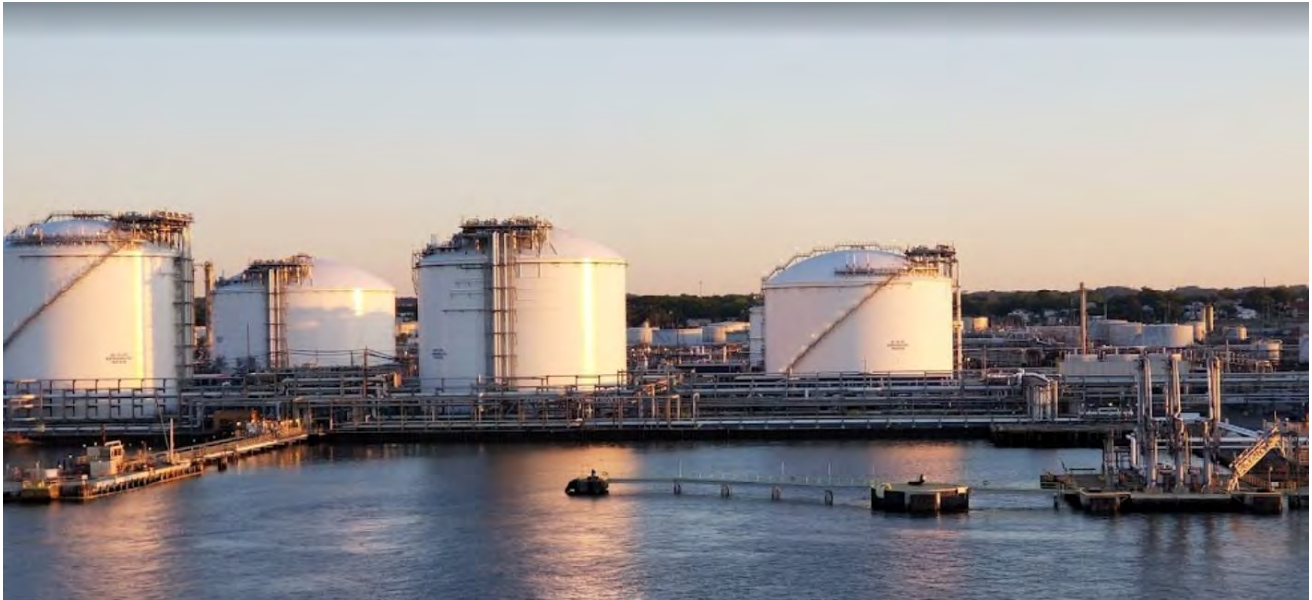
Figure 5: View of Marcus Hook Terminal Berths 3A (left), 3B (center) and 2A (right) (looking west).
