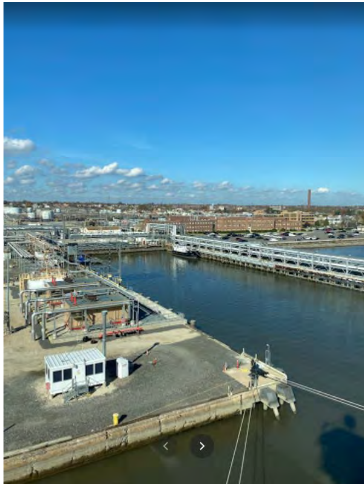
Figure 4: View of Marcus Hook Terminal Berths 2B, RW5, and 1B (looking west from in front of Berth 2A).
