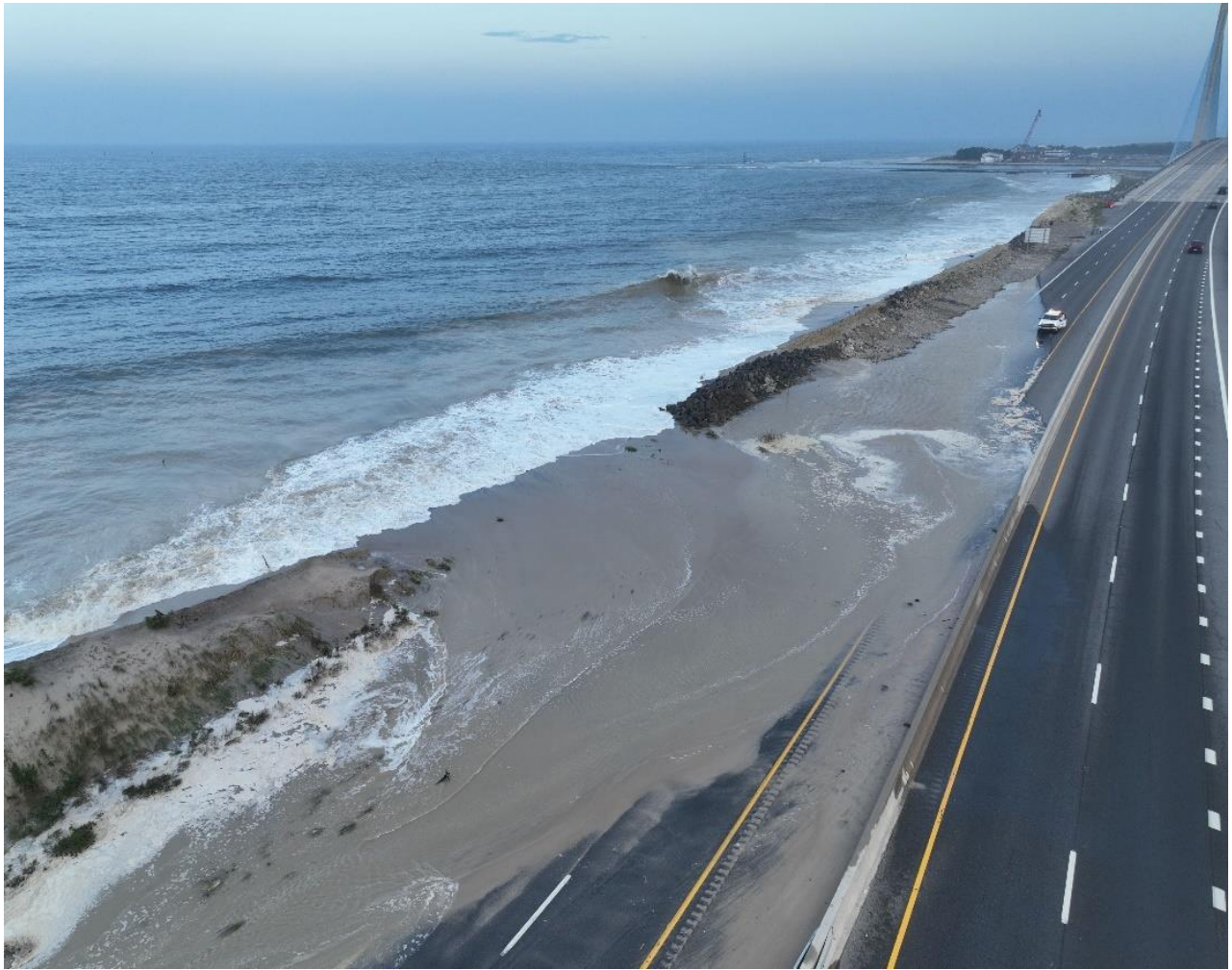
Figure 2. August 17, 2024. View of the dune breach at Delaware Seashore State Park (looking south). The SR-1 northbound lane is covered in water and sand, forcing a road closure.
