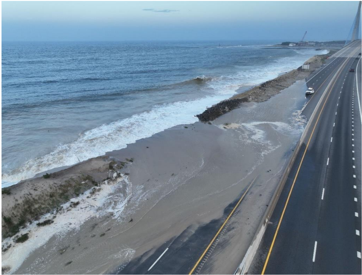
Photo 2. August 17, 2024. View of the dune breach at Delaware Seashore State Park (looking south). The SR-1 northbound lane is covered in water and sand, forcing a road closure.
