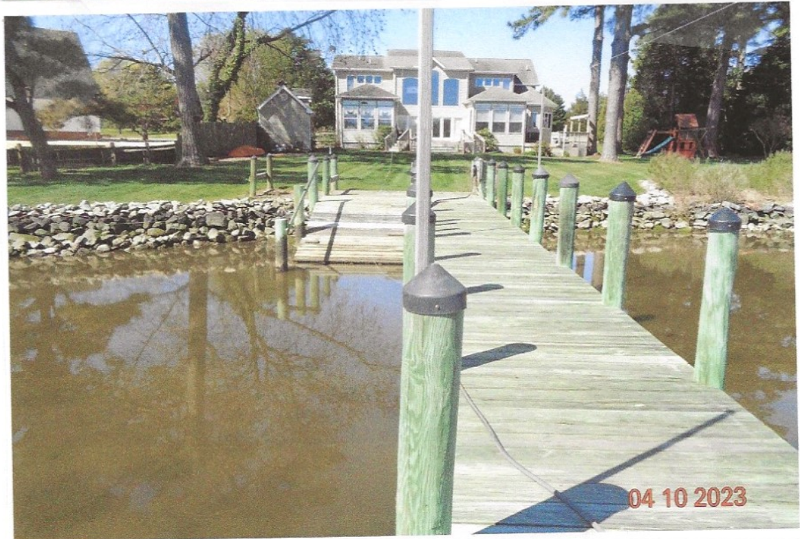
Figure 7. Ground-level photographs of site, 8 Sloan Road, Harbeson, Sussex County, Delaware (Tax Map Parcel # Parcel #2-34-17.12-96.00), adjacent to Burton Prong, Herring Creek (tributary of Rehoboth Bay). Applicant proposes to maintain existing structures (see Project Description for details), and to install 4 new free-standing mooring pilings. See Figure 8 for plan view and cross-section sketches.
