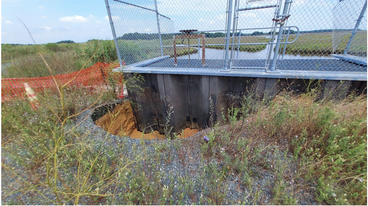
Figure 1: Damaged culvert due to subsidence (1 of 2)
