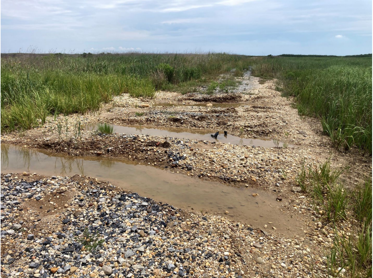
Figure 3: Failed section of existing levee to be repaired
