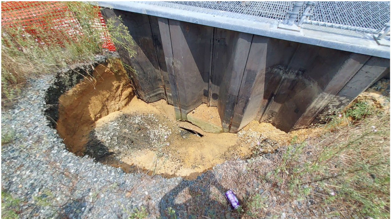
Figure 2: Damaged culvert due to subsidence (2 of 2)
