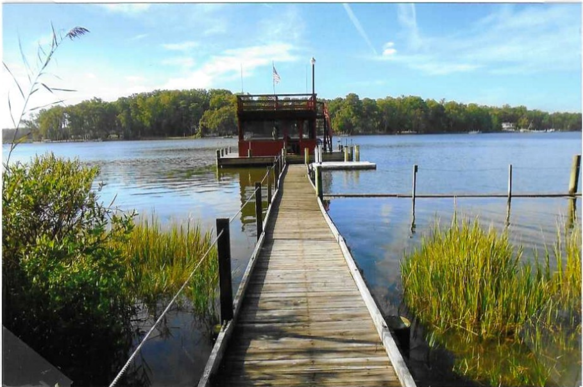
Figure 7. Ground-level photograph of site, 23392 Angola Beach Road, Lewes, Sussex County, Delaware (Tax Map Parcel #234-18.00-6.00), adjacent to Herring Creek (tributary of Rehoboth Bay). Existing structure consists of a walkway/pier, 70' long (channelward of MHWL) x 5.5' wide; a finger pier 22.5' long x 3.5' wide; and a platform 20' long x 24' wide with a 12' long x 14' wide gazebo and rooftop observation deck. Structure was constructed in 1968 (grandfathered), see Figure 6b for 1968 aerial photograph. A 12'± long x 4.5±' wide floating PWC dock was installed at a later date. Applicant proposes to repair/replace/elevate (by 18") the pier and finger pier; and seeks authorization for the PWC dock. See Figure 8 for plan view and cross-section sketches.
