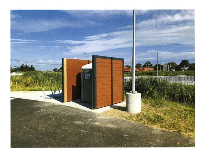
Figure 2. Example of a three-sided porta potty enclosure.
