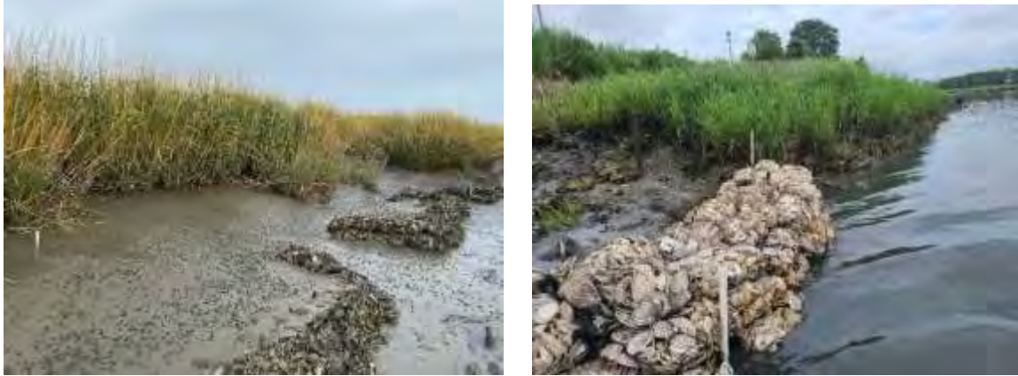
Figure 8. Shell bags installed as part of a living shoreline at Mispillion (left) and Lewes Ball Field (right).
