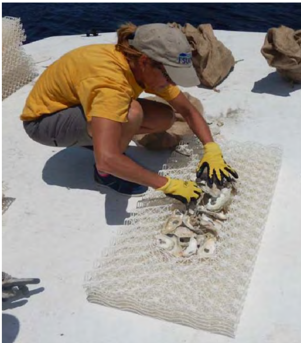
Figure 4. BESE-ELEMENTS® Biodegradable ecosystem engineering elements secure mixed shells in the lower energy environment.
