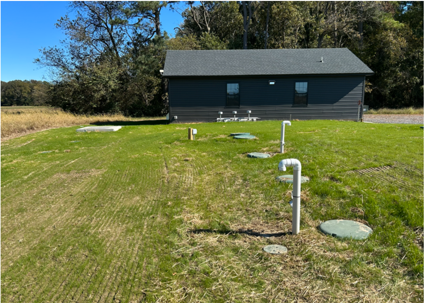
Photo #3 - Showing the Wastewater Treatment Building and the Vent Pipes Coming from the Tanks (side view)
