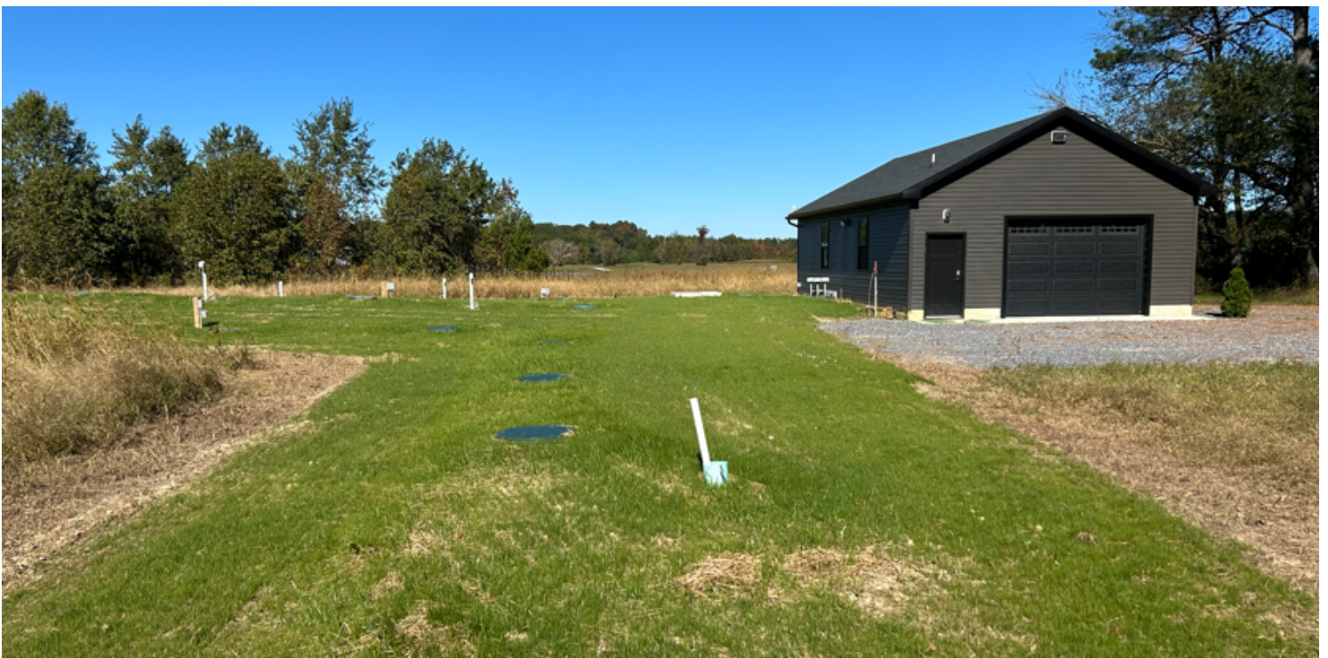
Photo #2 - Showing the Wastewater Treatment Building and the Vent Pipes Coming from the Tanks.
