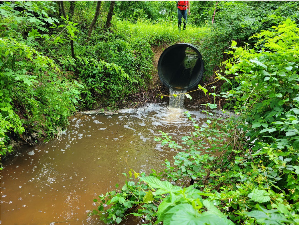
Photograph 2: View of existing culvert outfall.
