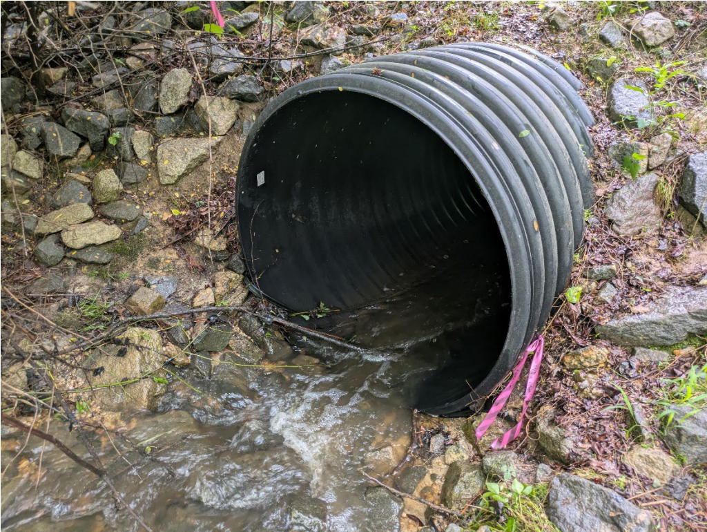
Photograph 1: View of existing culvert inlet.
