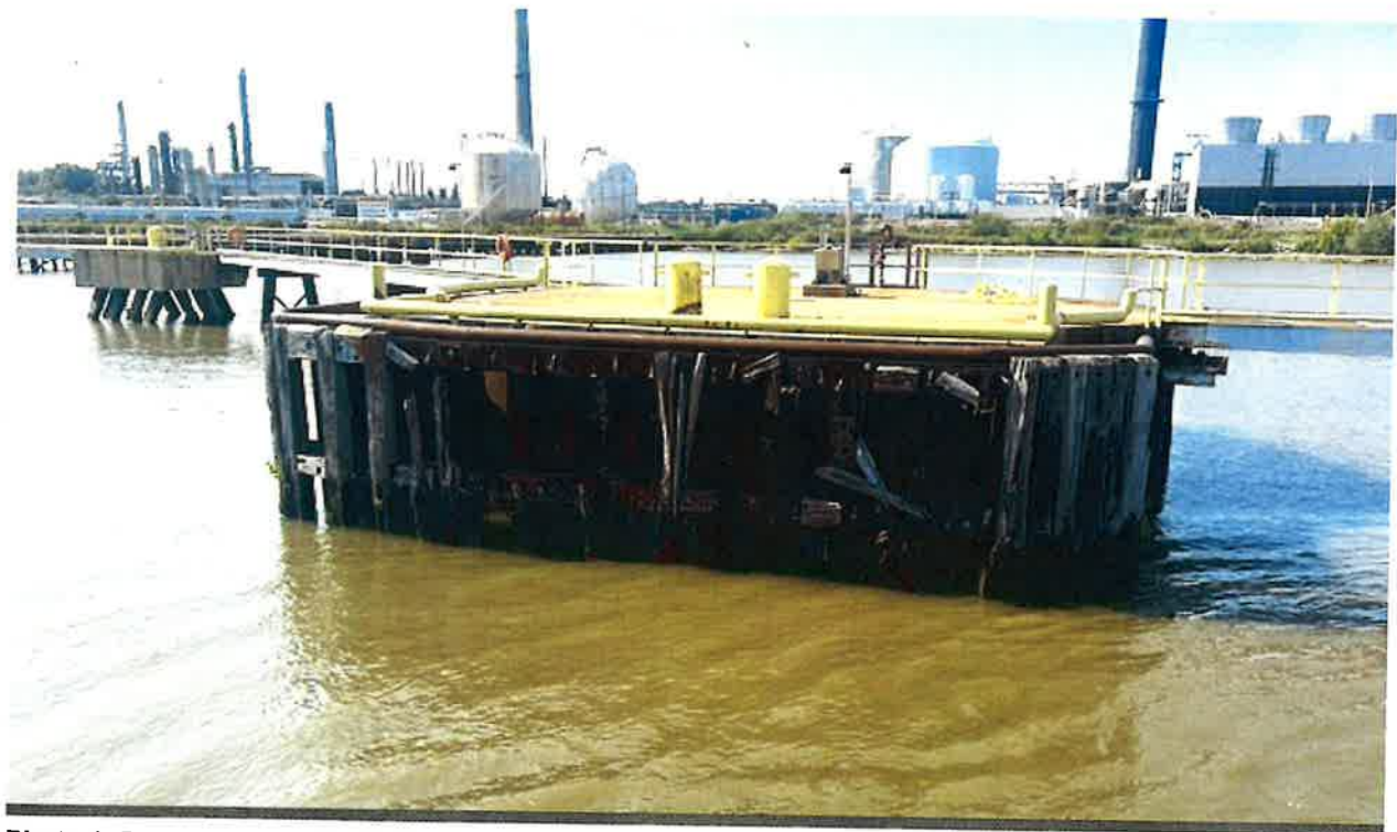
Photo 1: Downriver Breasting Cell.
