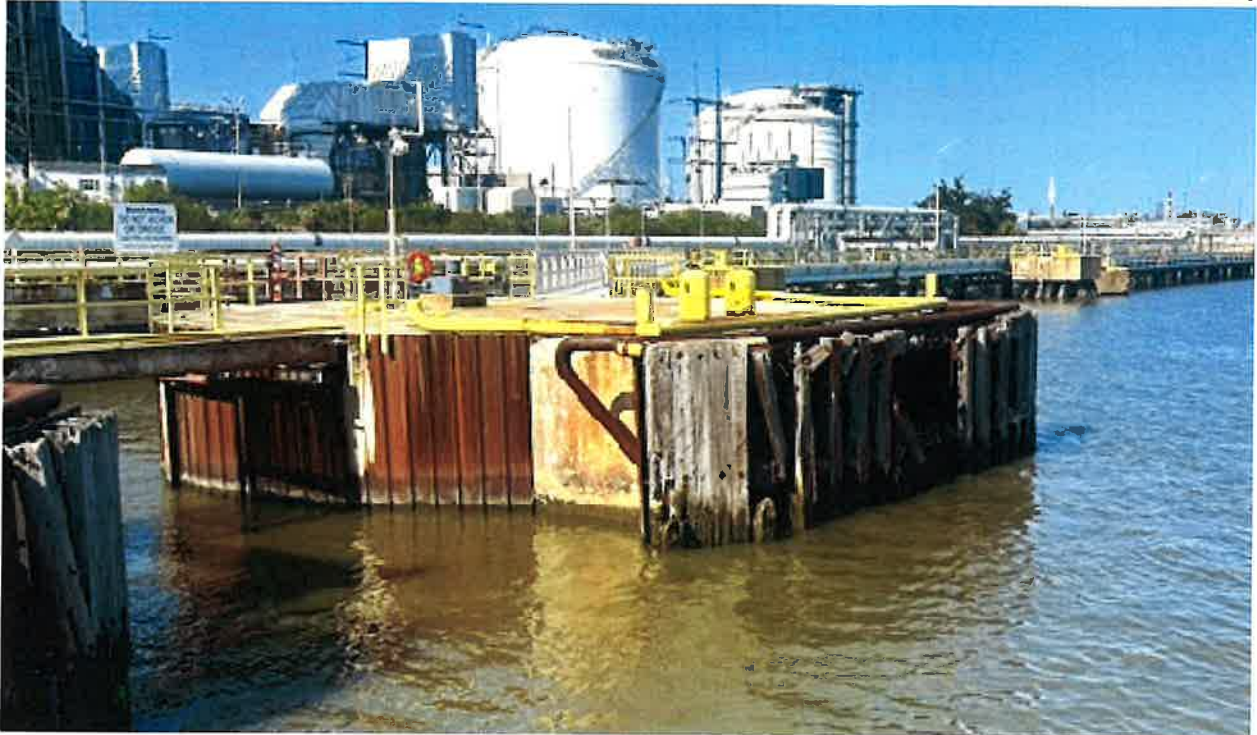
Photo 2: Upriver Breasting Cell.
