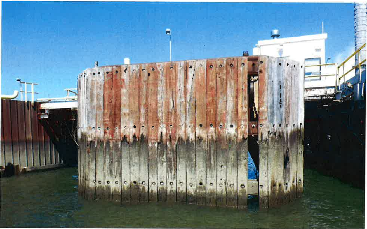
Photo 3: Downriver Breasting Dolphin.
