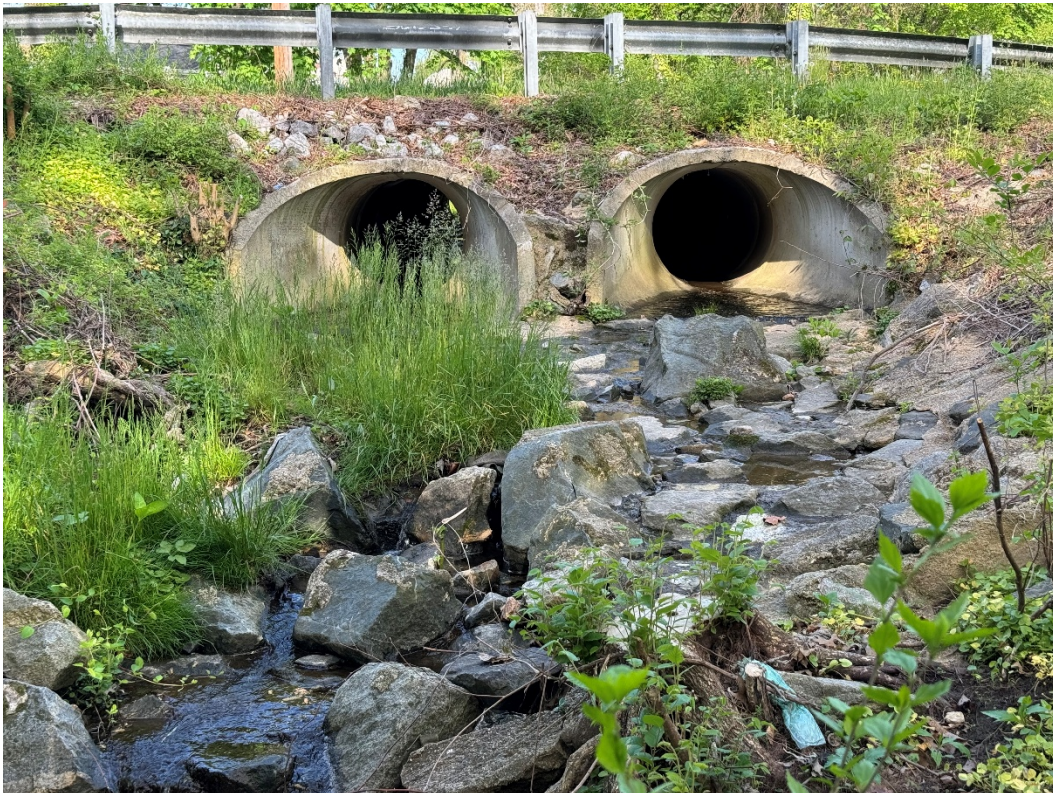
Photo 2: Outfall of twin 42-inch RCPs below Armstrong Avenue
