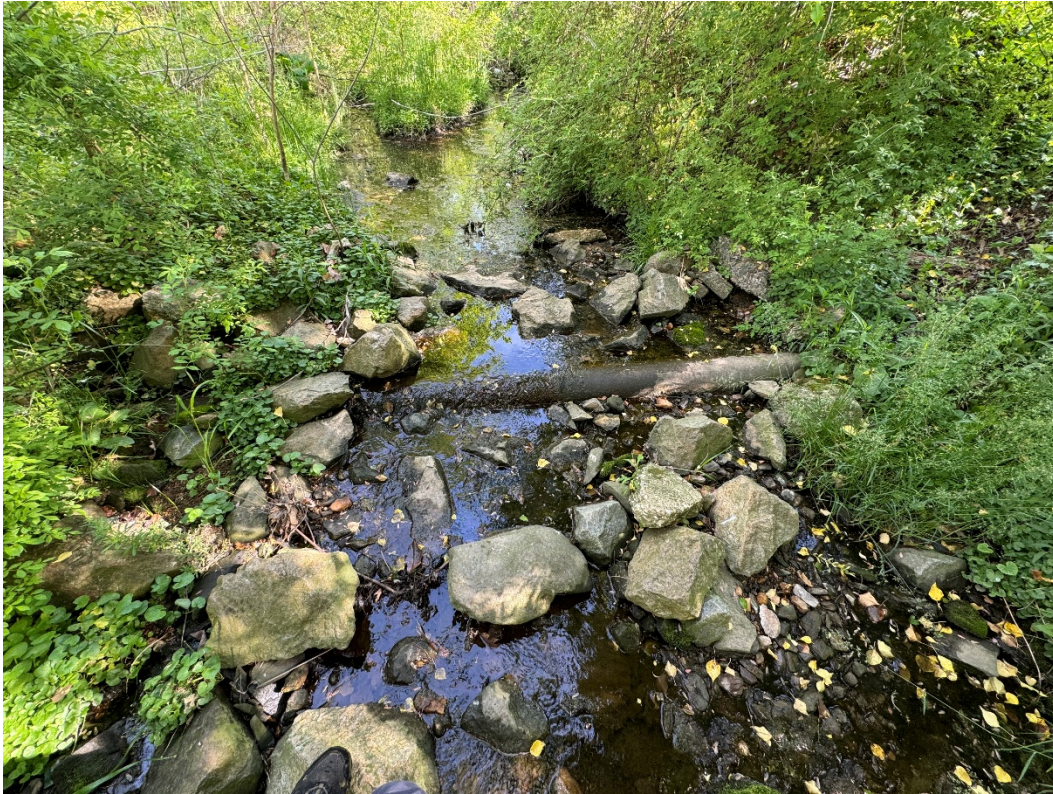
Photo 1: Exposed sewer in existing channel
