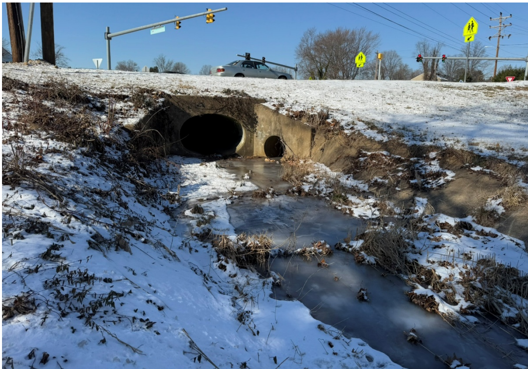
PHOTO 8: OUTFALL 1A AND 1B
