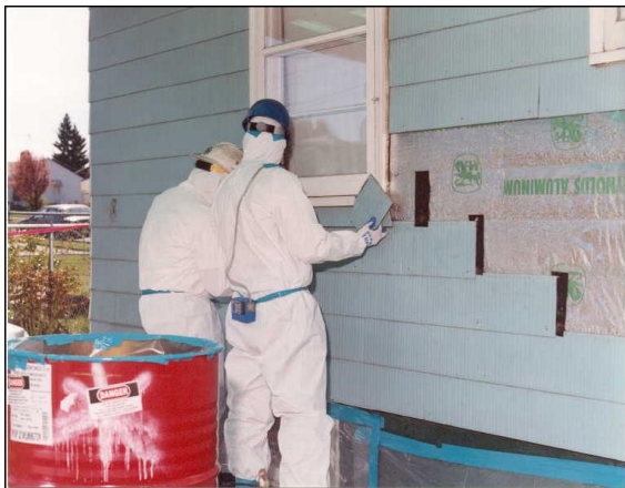
Removing siding
