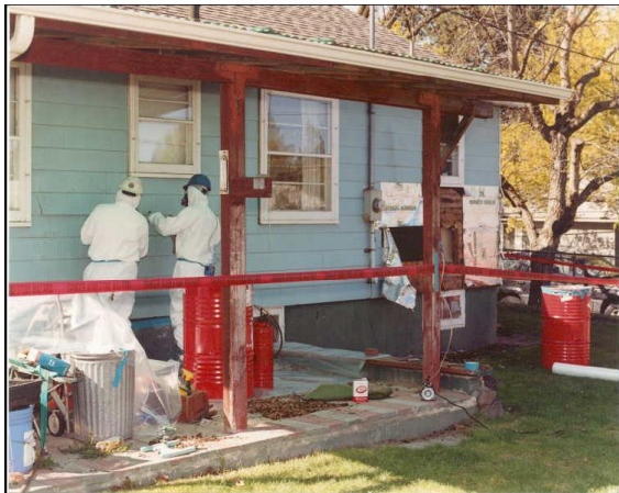
Prying to expose nail heads
