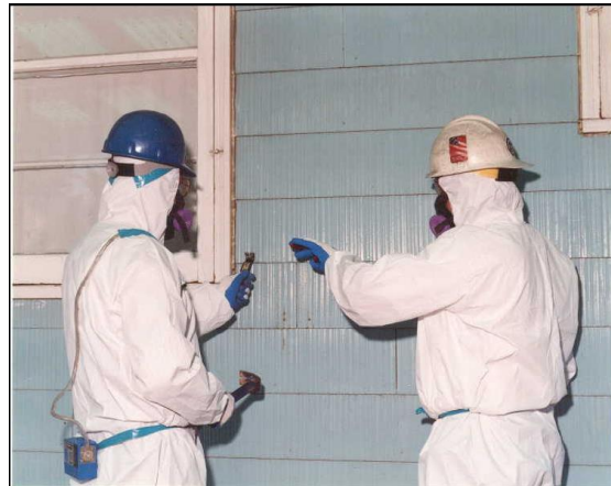
Pulling out nails
