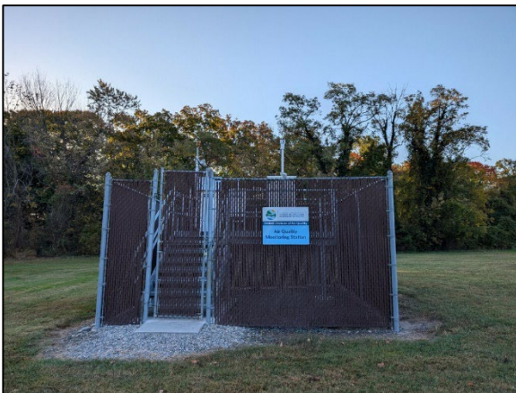
Dover Monitoring Platform
