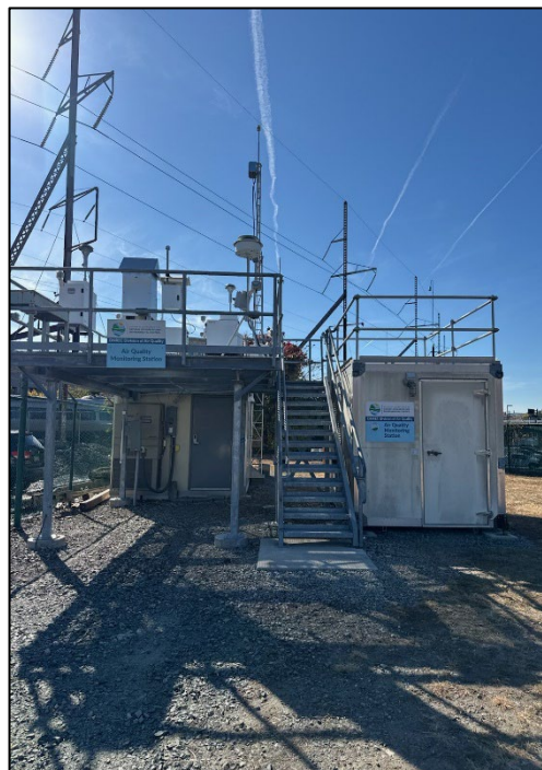
MLK NCore Station
