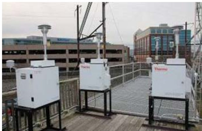
Particulate Monitoring at MLK NCore
