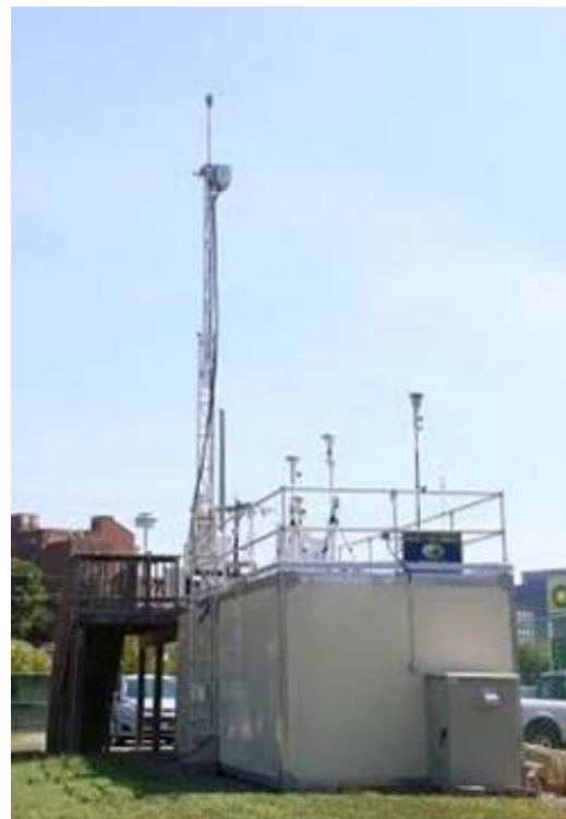
MLK NCore Station
