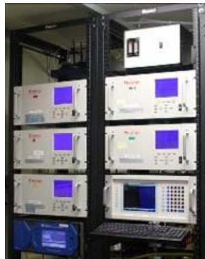
MLK NCore Criteria Gas Analyzers
