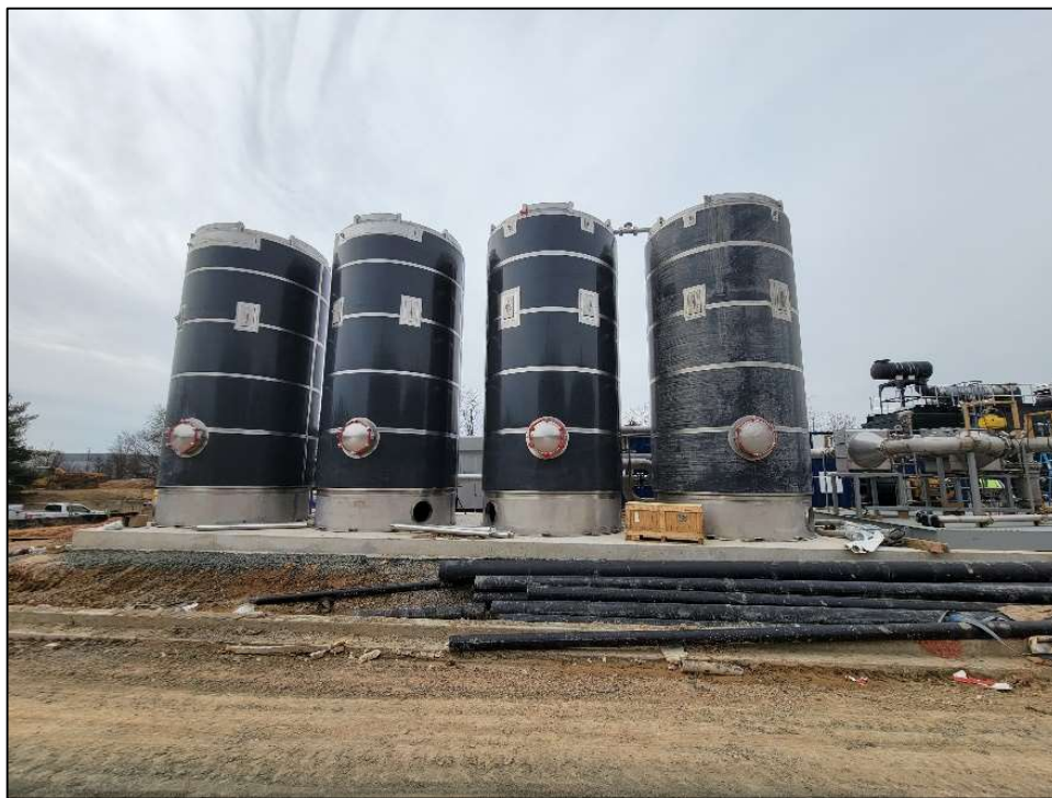
Figure 25: H 2 S and VOC/Siloxane Removal Vessels at Jessup, MD Facility
