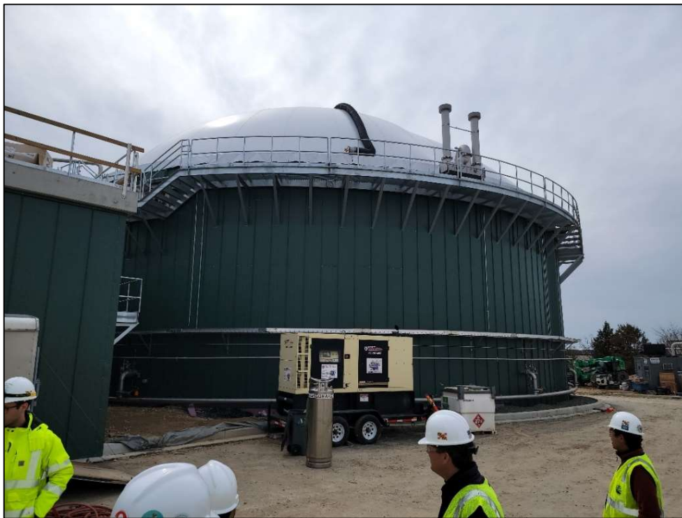
Figure 14: Digester at BioEnergy Jessup, MD Facility
