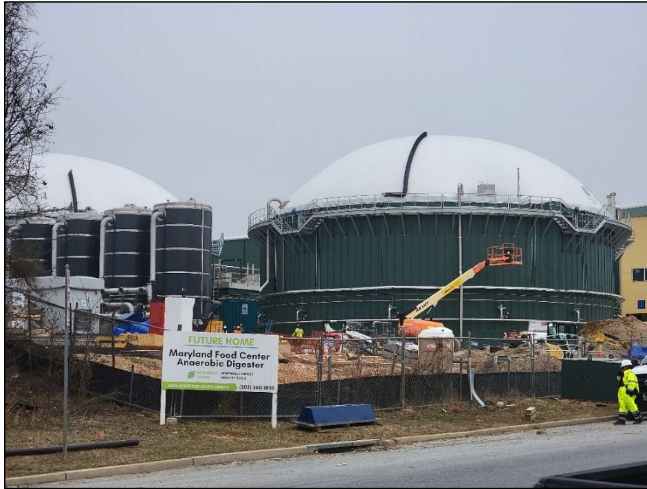
Figure 13: Digester at BioEnergy Jessup, MD Facility
