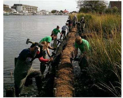
**LEWES CANAL LIVING SHORELINE** The goal of the Lewes Canal living shoreline is to protect the property from further erosion due to boat wake and wave energy and prevent the eroding sediment from building up in the canal. The project structures, including coconut fiber coir logs, coconut mats, and oyster shell bags, were installed in April 2014 and planted in April 2015.
