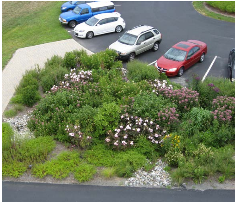
RAIN GARDEN, UD LEWES CAMPUS The rain garden at the University of Delaware's Hugh R. Sharp Campus in Lewes was designed to provide infiltration of surface water runoff from the adjacent parking area. The garden was installed in 2010 with assistance from Delaware Sea Grant and DNREC.
