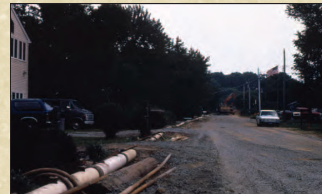
Sanitary sewer lines being installed, part of the wastewater infrastructure in the basin
