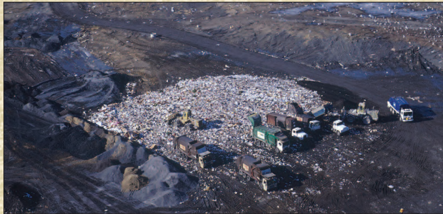
The Delaware Solid Waste Authority's Cherry Island Landfill; located along the Delaware River in New Castle County
