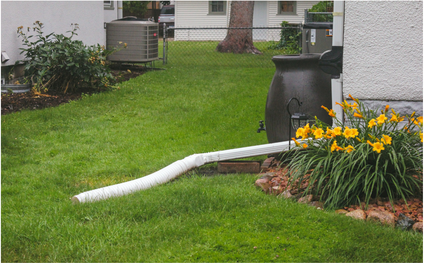
Residential downspout extension and rain barrel (Source: flickr, Mississippi Watershed Management Organization, CC BY-SA 2.0)
