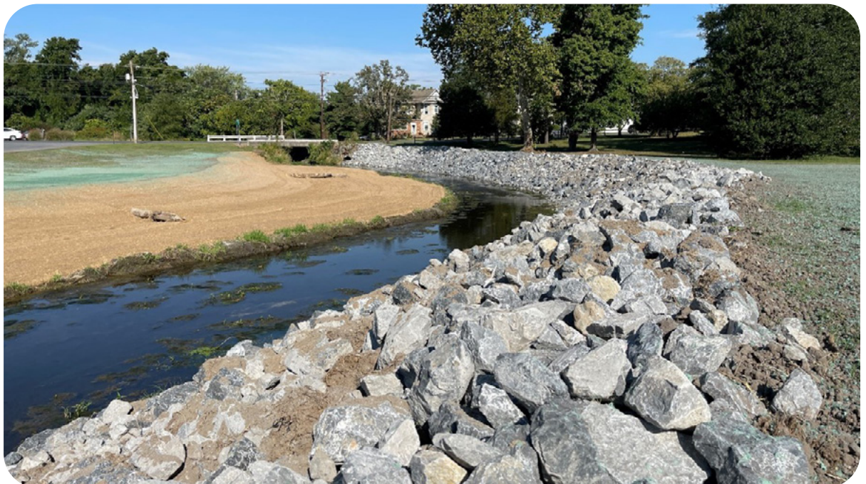
Completed Restoration – Floodplain Expansion, Stabilization and Channel Bottom Dip Out (Looking West)
