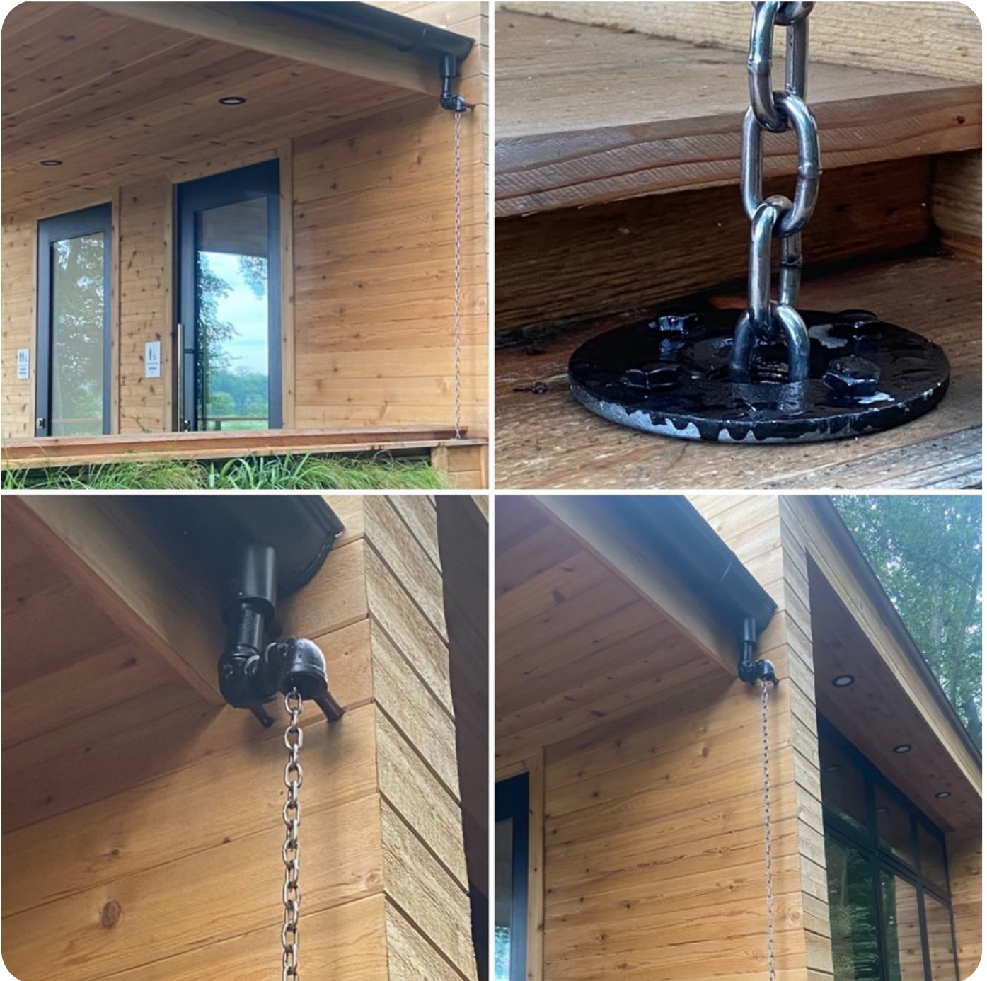
Rain Chains Directing Rooftop to Living Wall for Stormwater Recycling
