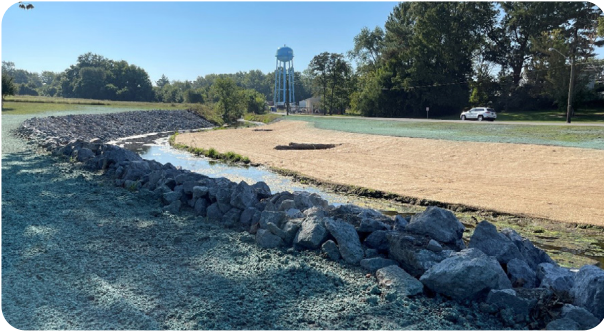
Completed Restoration – Floodplain Expansion, Stabilization and Channel Bottom Dip Out (Looking East)
