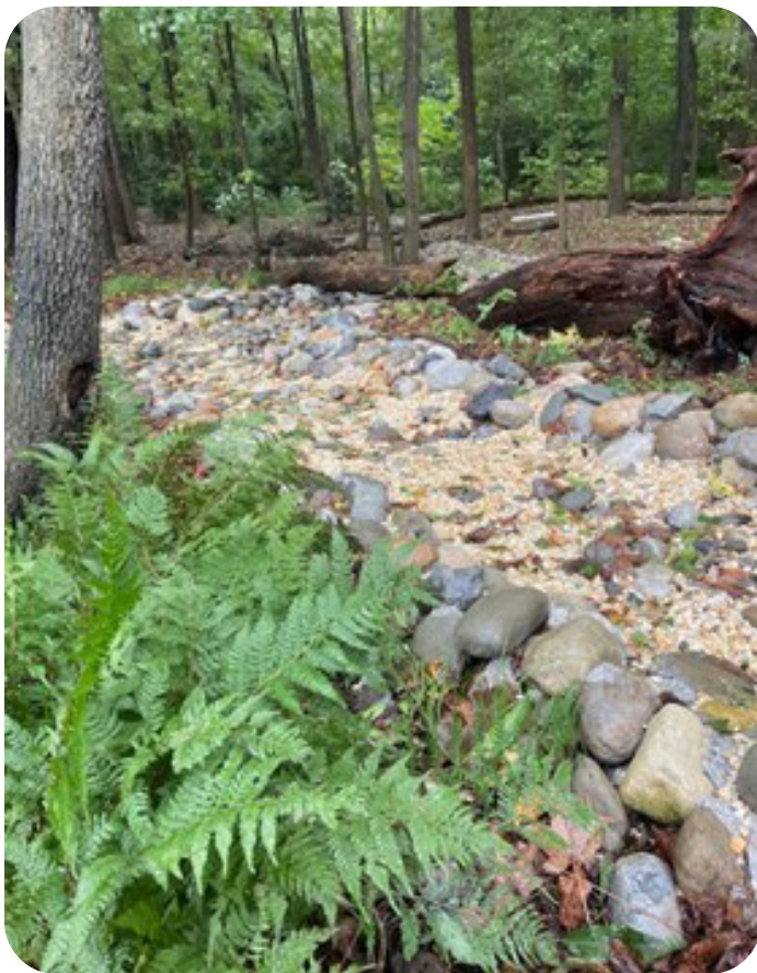
River Rock Channel Directing Stormwater Runoff to Vernal Pool
