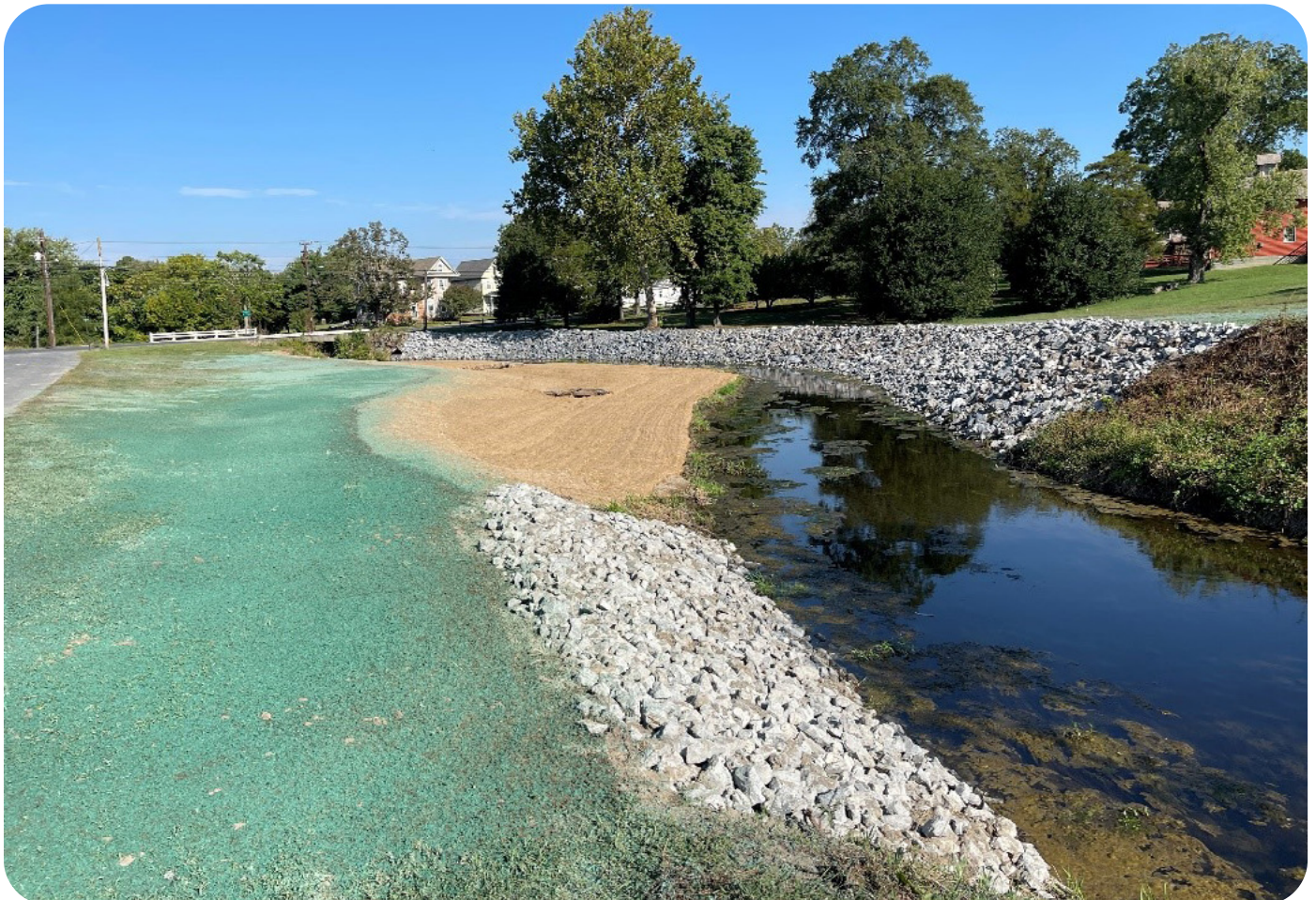
Completed Restoration – Floodplain Expansion, Stabilization, and Channel Bottom Dip Out (Looking West)
