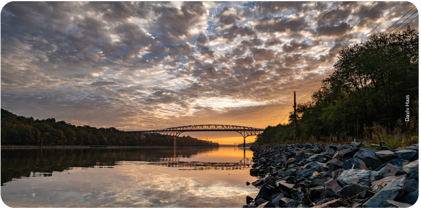
South side of the C&D Canal, west of Summit Bridge
