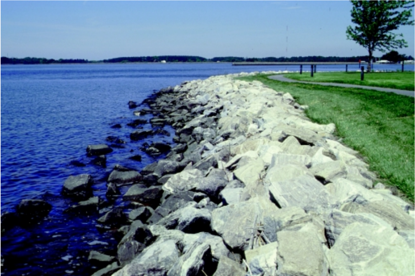
Figure 16-51 Rock riprap revetment
