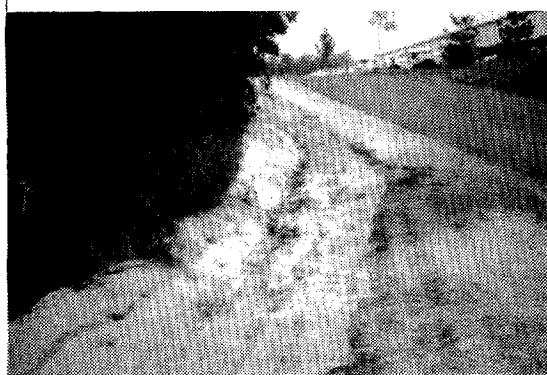
Figure 8. Installed Woven Paper Net Lining.
