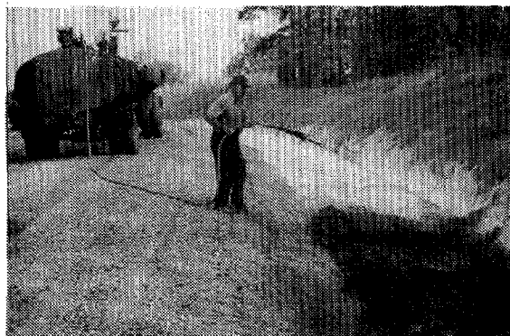
Figure 12. Installation of Fiberglass Roving Along a Roadside.
