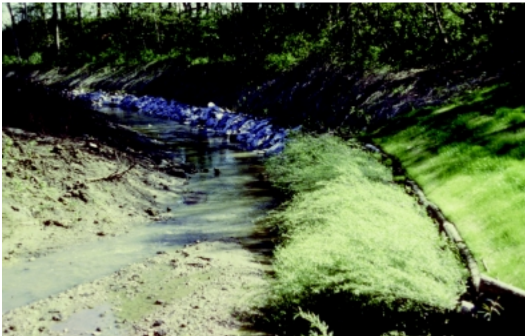
Figure 16-15c An established live cribwall system
