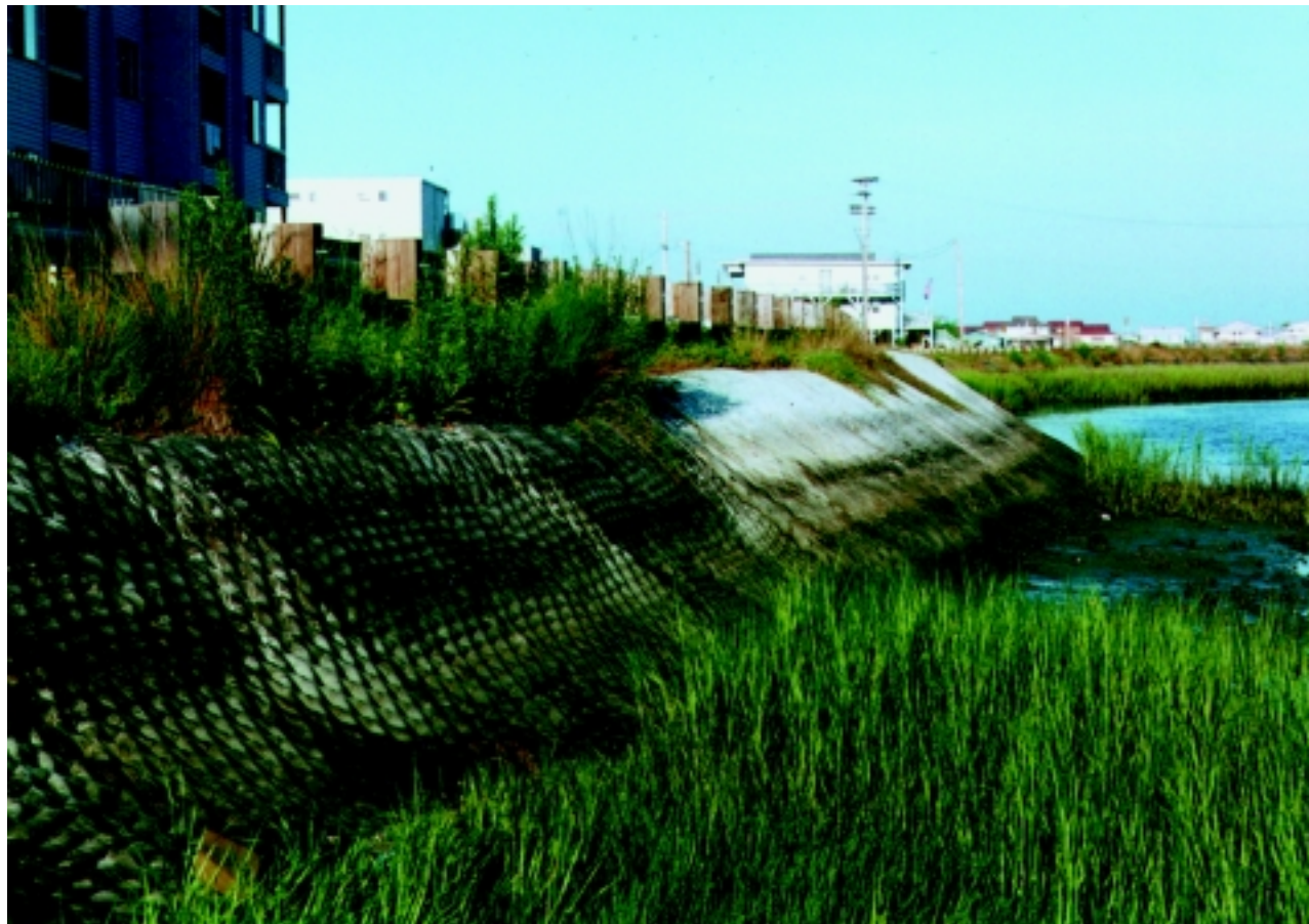
Figure 16–50 Concrete revetment (poured in place)
