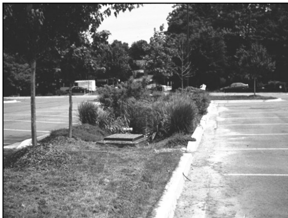
Figure 2: Parking Lot Island Turned Bioretention Area
