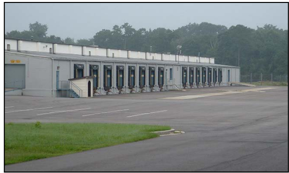
Figure 1: Loading/Unloading Area of Warehouse
