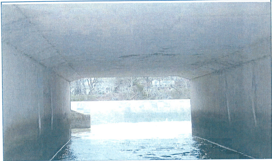
3. GENERAL VIEW (LOOKING WEST THRU S. CELL)
