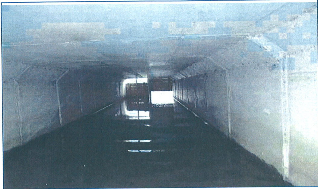
3. GENERAL VIEW (LOOKING WEST)
