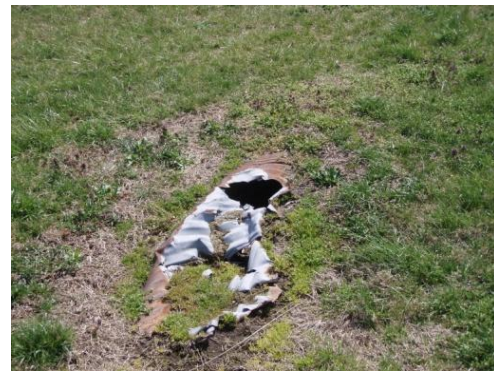
Completely collapsed culvert on Southbound Route 13 at Herr's Foods
