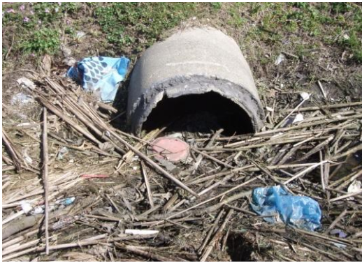
Outfall on northbound Route 13 on the property south of Food Lion
