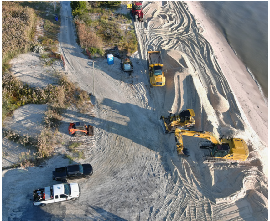
Pickering Beach project during construction
