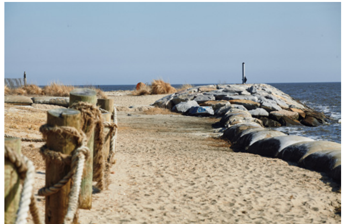
Bowers Beach jetty along the Murderkill River Inlet
