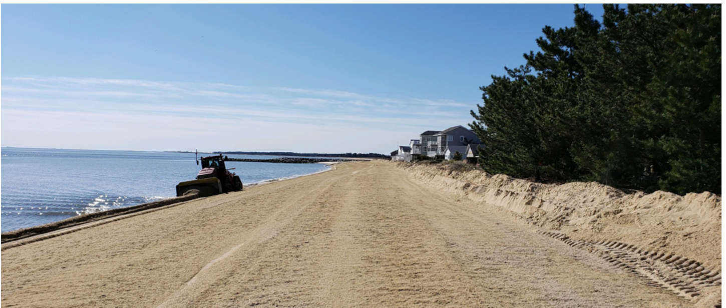
Beach nourishment project in progress.
